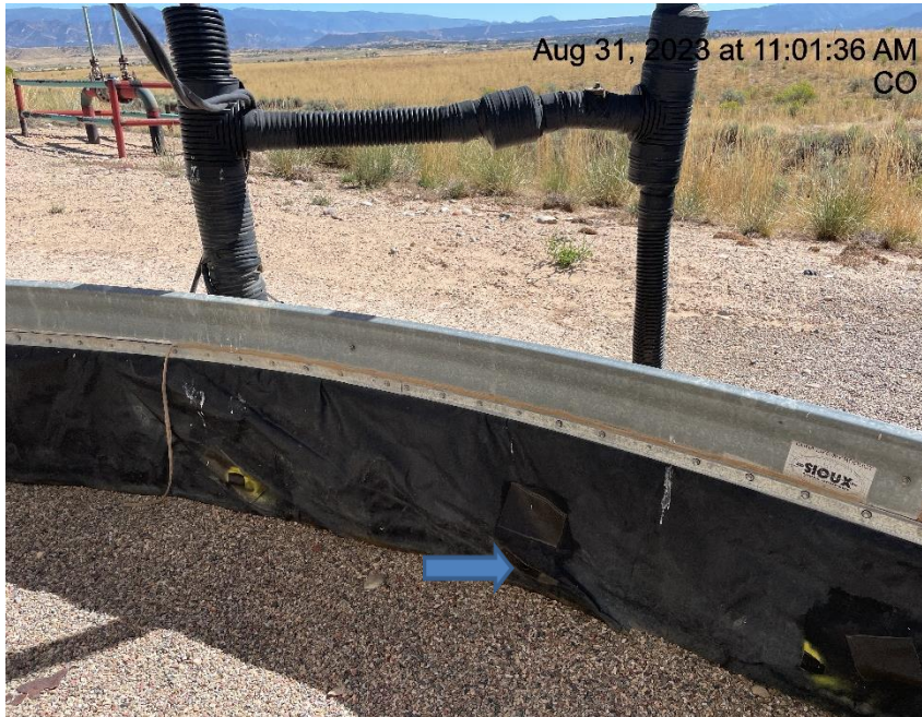
Photo # 7853 Hole in liner/liner needs maintenance
