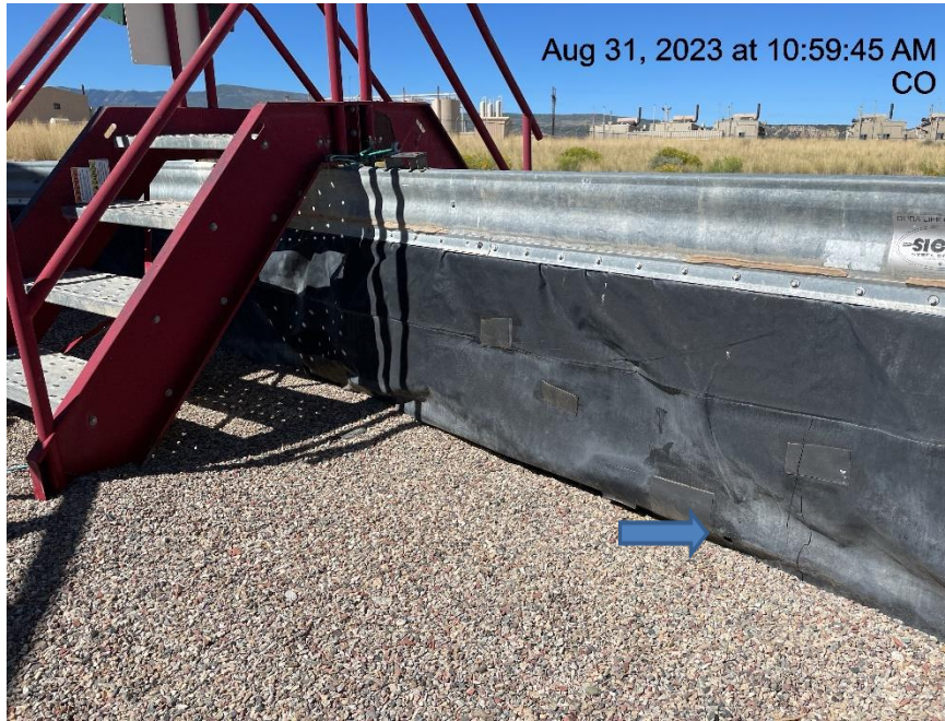
Photo # 7848 Hole in liner/liner needs maintenance
