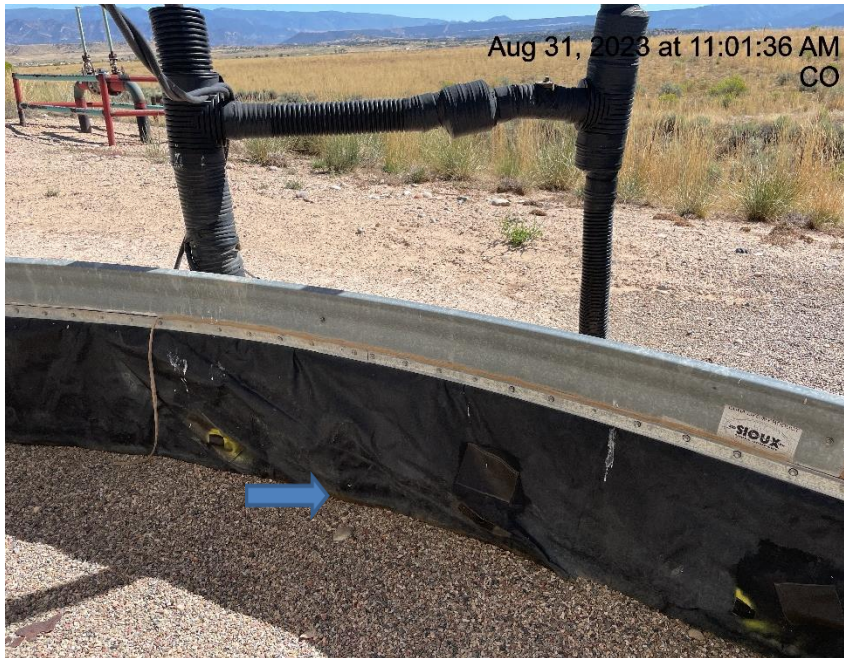
Photo # 7853 Holes in liner/liner needs maintenance
