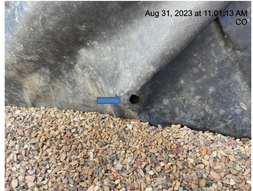
Photo # 7852 Hole in liner/liner needs maintenance
