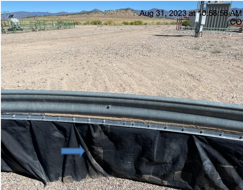
Photo # 7844 Hole in liner/liner needs maintenance
