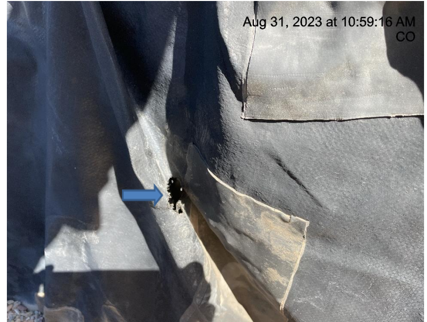
Photo # 7846 Hole in liner/liner needs maintenance
