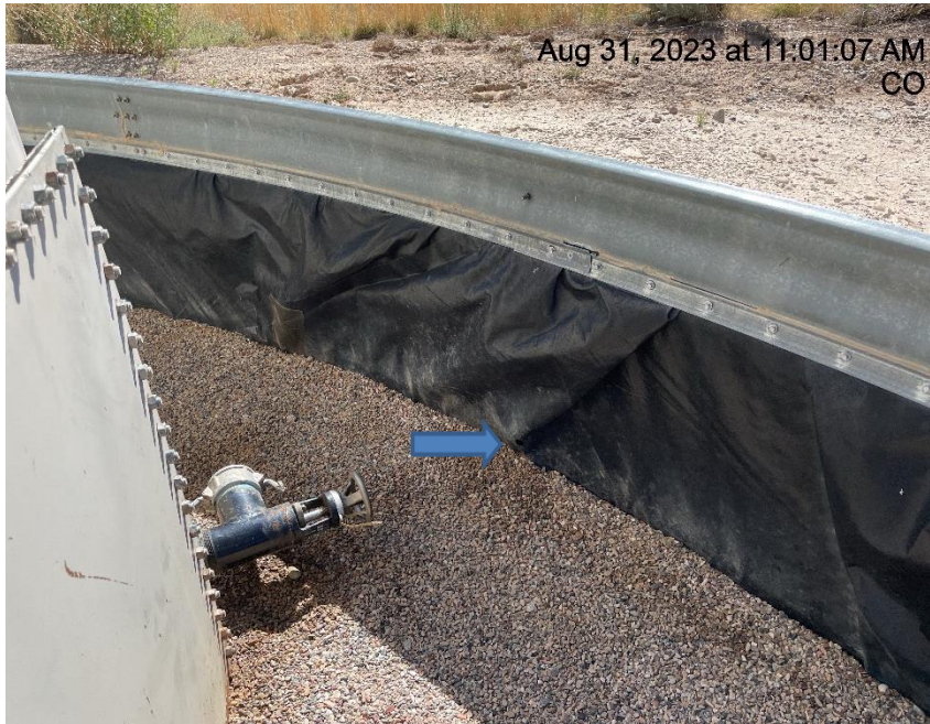
Photo # 7851 Hole in liner/liner needs maintenance
