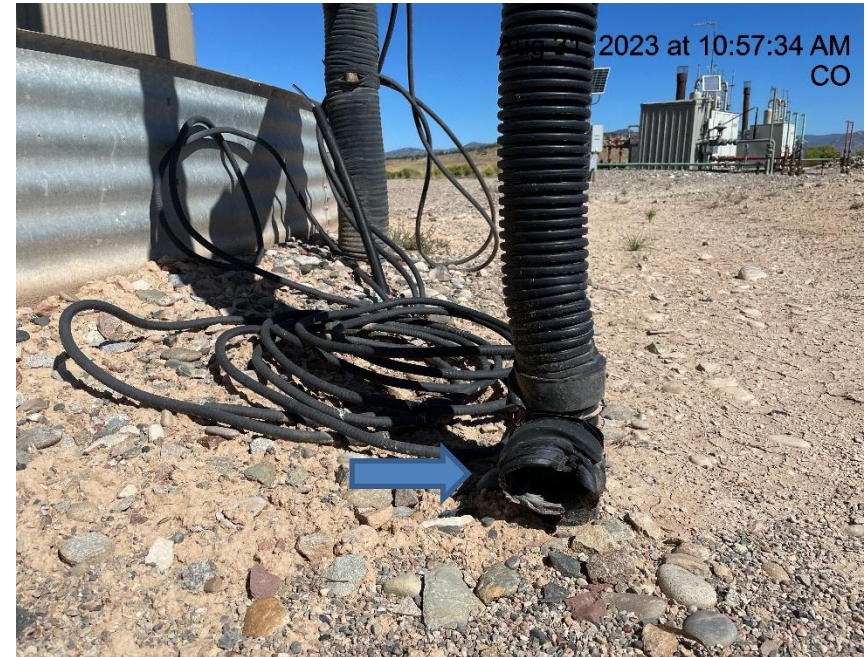
Photo # 7843 Flowline heating insulation open ended
