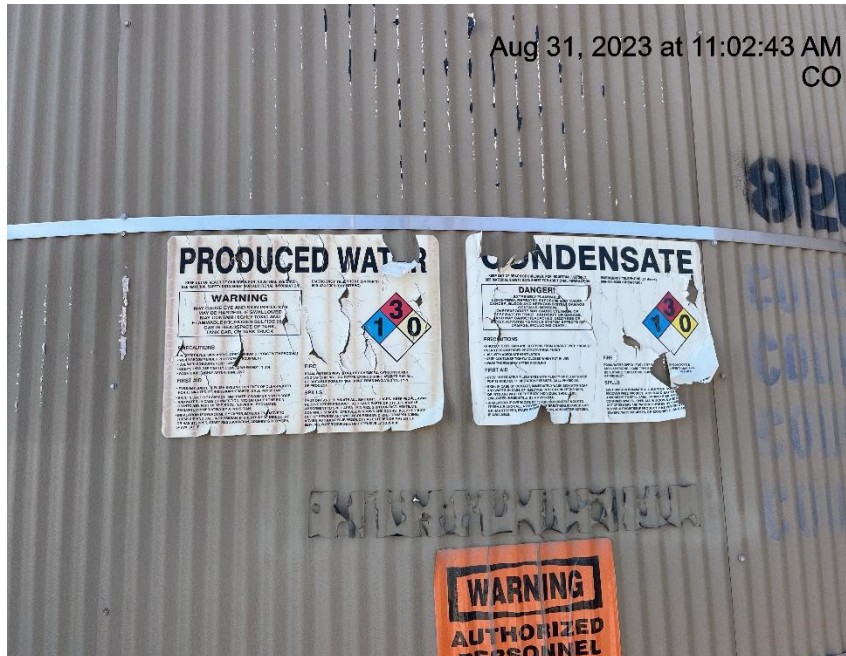
Photo # 7858 Tank labels peeling off
