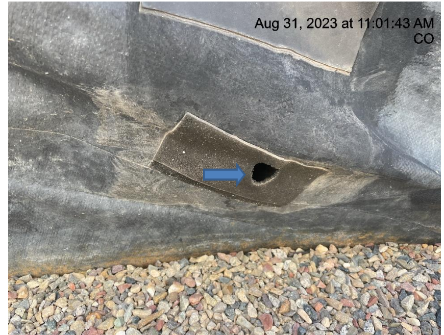
Photo # 7854 Hole in liner/liner needs maintenance
