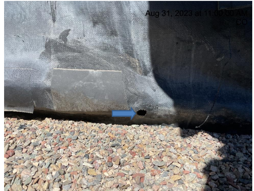
Photo # 7849 Hole in liner/liner needs maintenance
