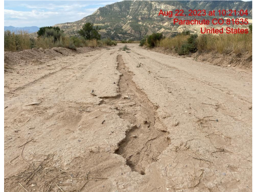
Rill Erosion on Access Road – Photo #06013
