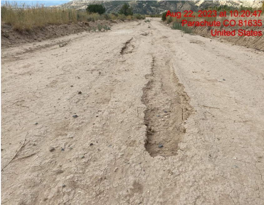
Rill Erosion on Access Road – Photo #06012
