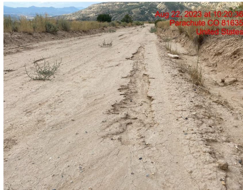
Rill Erosion on Access Road – Photo #06011
