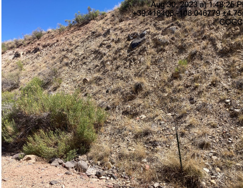
Some areas of cut slope show signs of erosion and lack of stabilization
