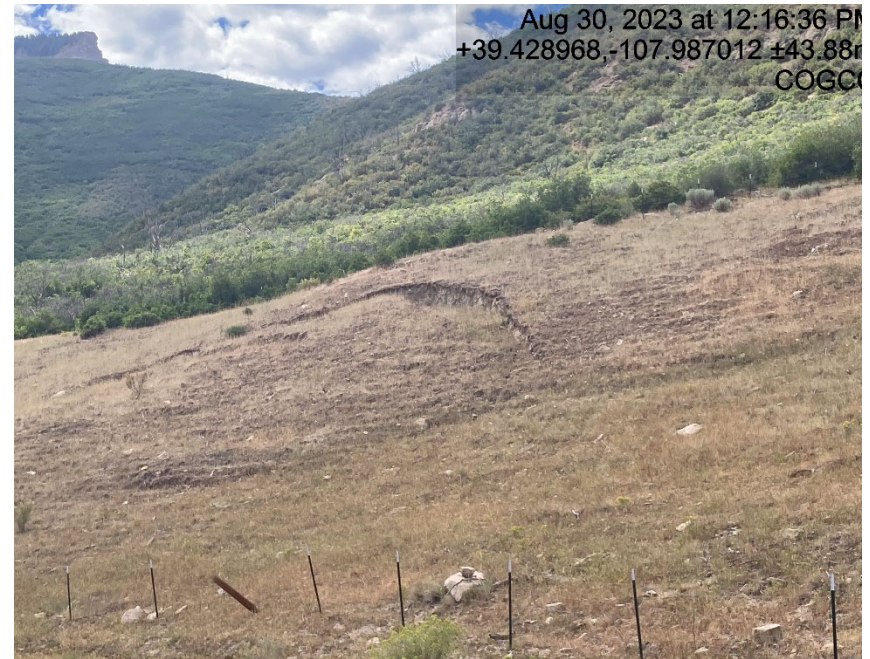
Cut slope is sluffing
