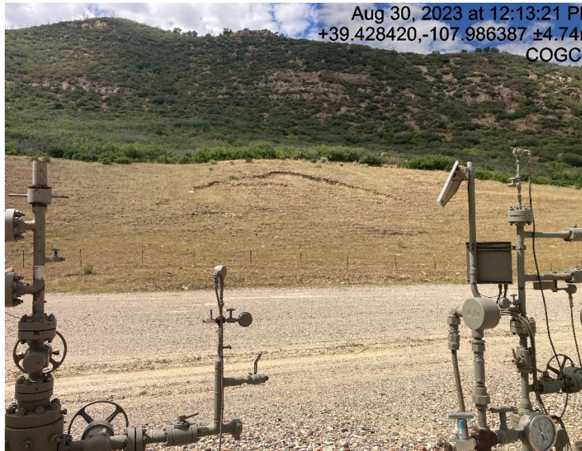
Cut slope is sluffing
