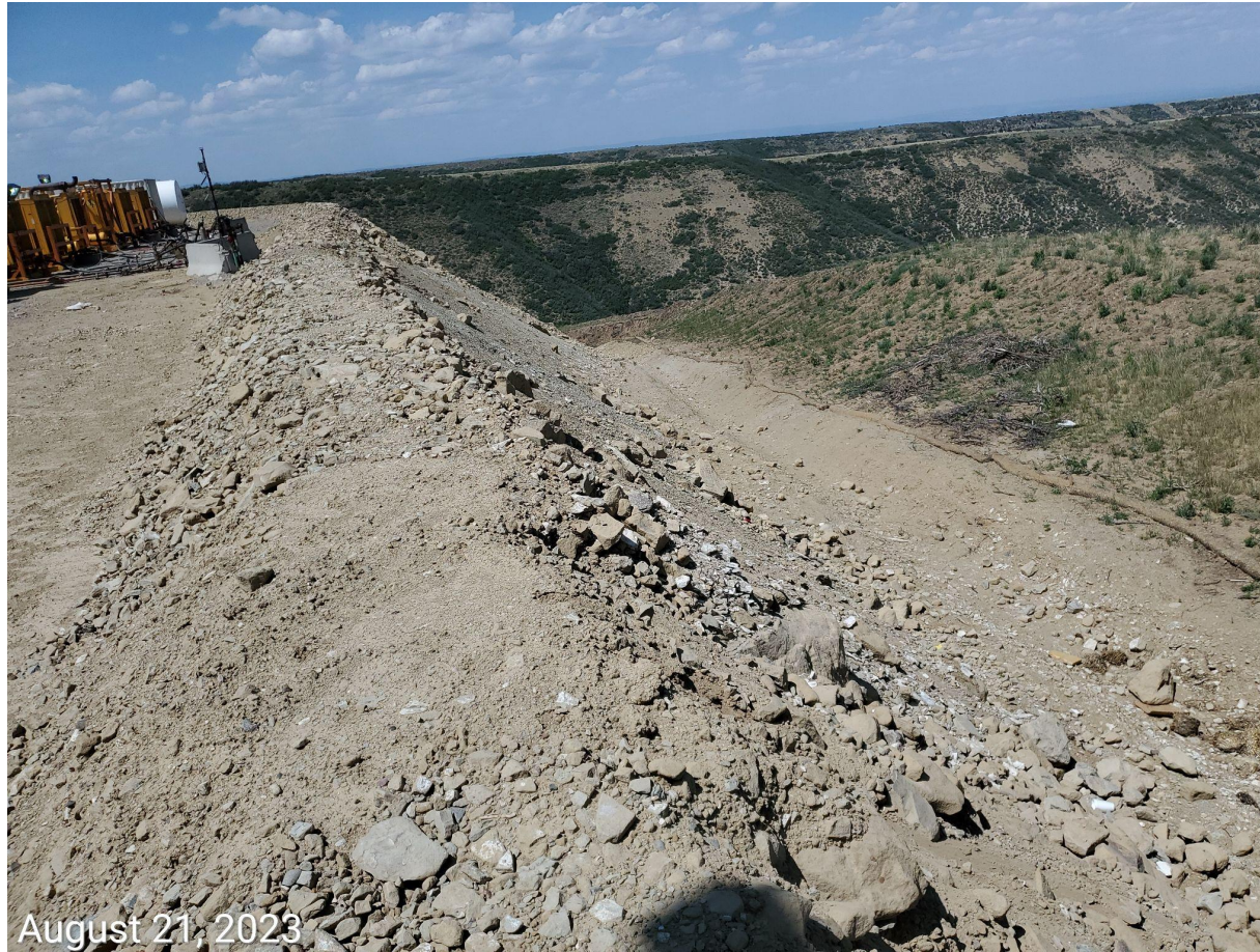
Photo 7: Stormwater ditch. BMPs per the Location Drawing / SWMP not observed.
