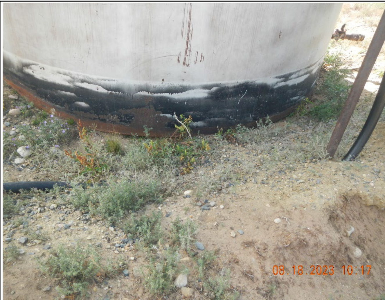
Photo #13 Poly line is buried in the tank Berm.
