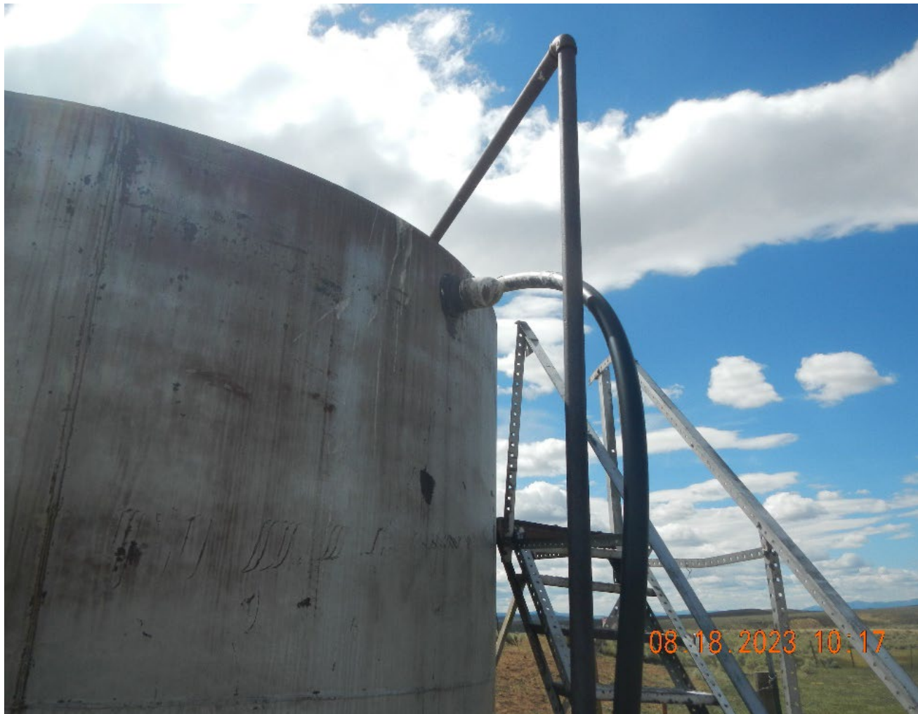
Photo #14 Poly line entering the Production Tank.
