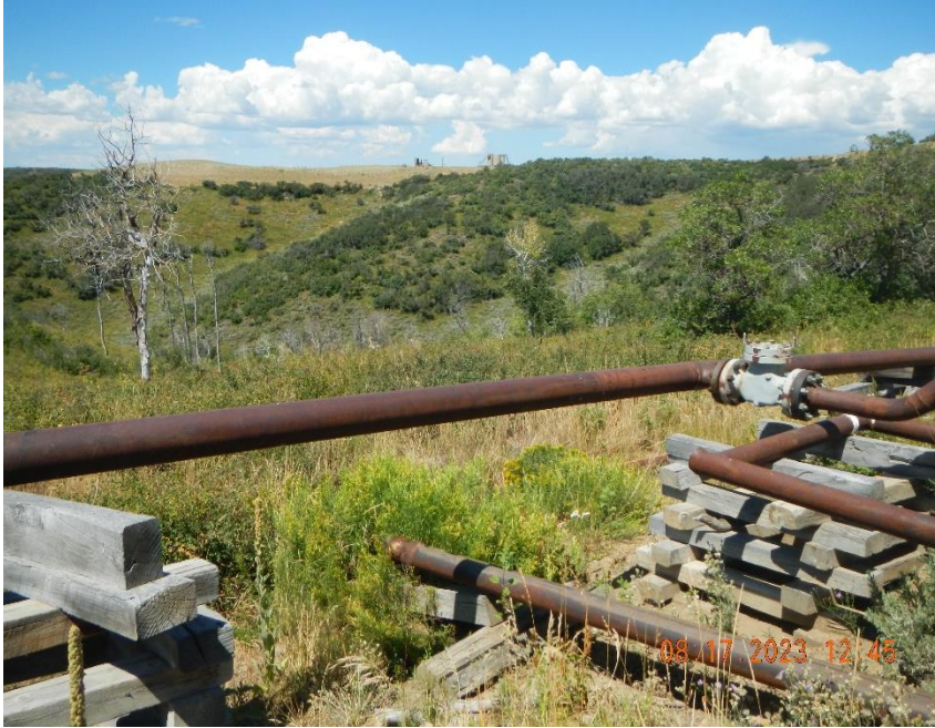
2- 4" flowlines running to the east under the road
