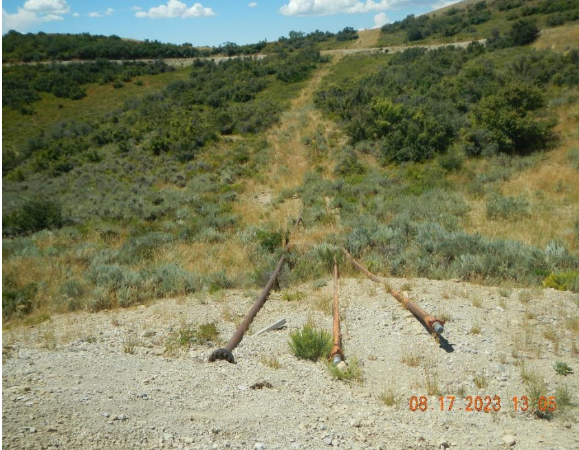
Unused flowlines leaving west side of location of Pond G.
