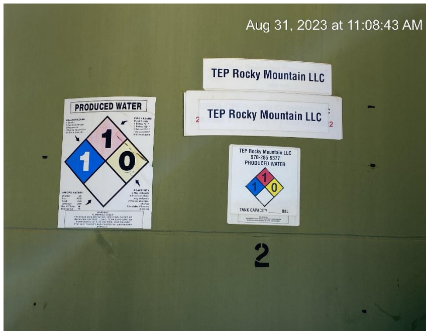
Missing tank capacity information
