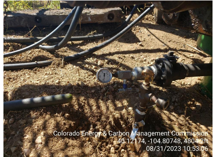
Photo 6 Casing pressure gauge at 400 psi. post test.
