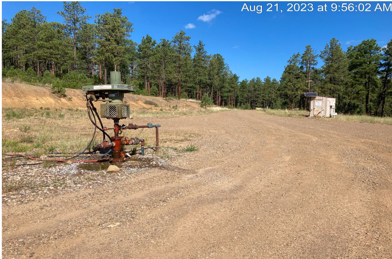
Photo 2. Facing toward the well. There is a dripping leak at the wellhead.
