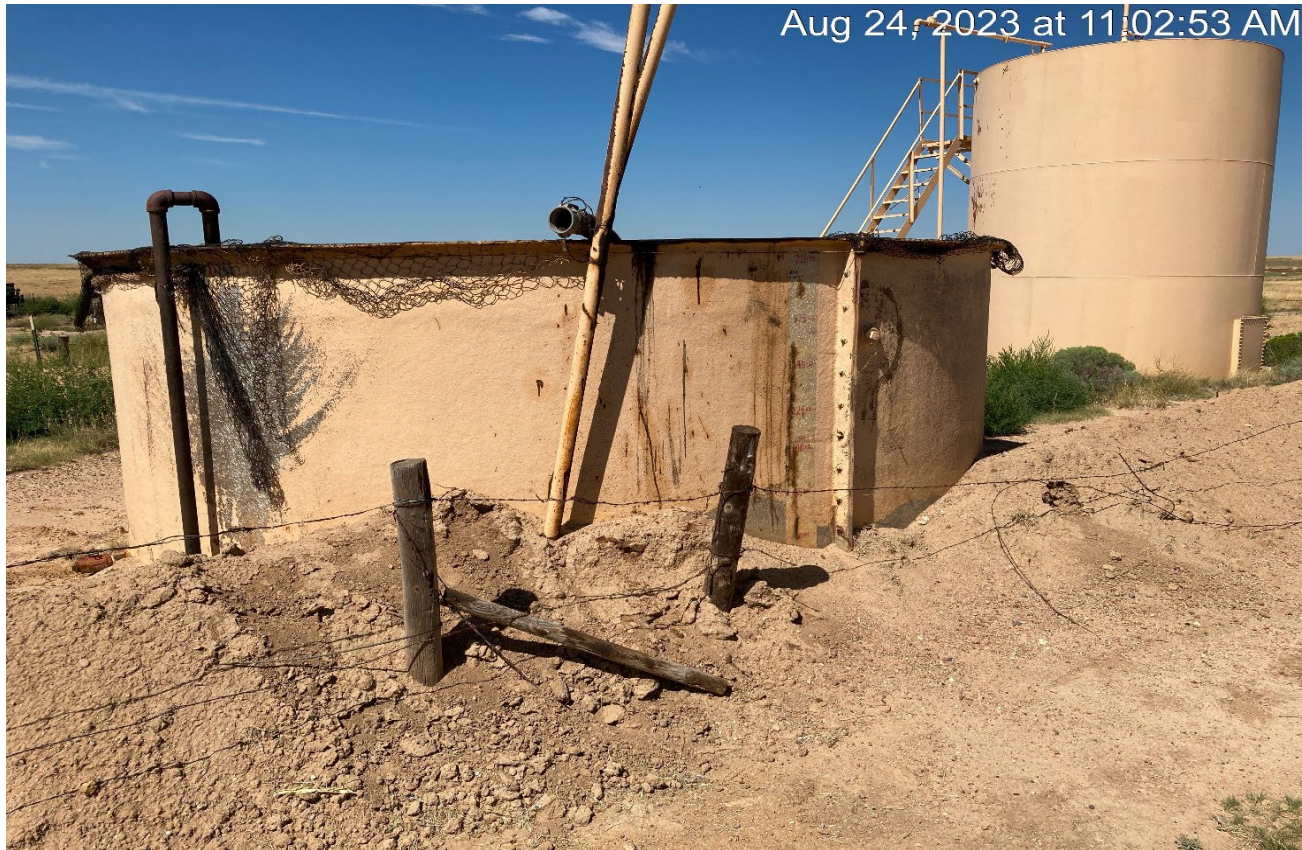
Photo 5. The berm is inadequate to contain a spill as it is piled up against the tank and would spill over the berm along this side. Previous corrective action was not completed.
