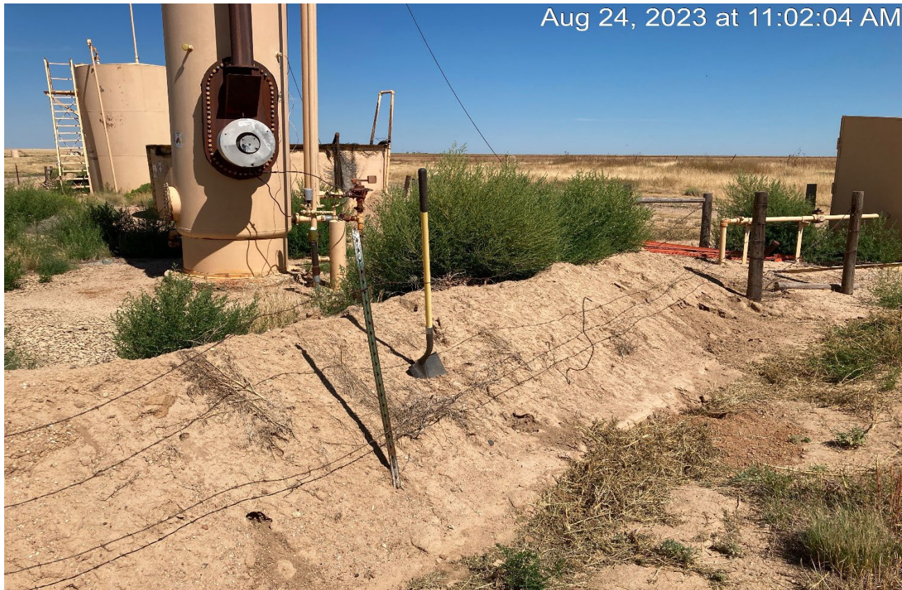
Photo 4. The fence around the tank battery is inadequate to prevent livestock entry and is not maintained. Previous corrective action was not completed.
