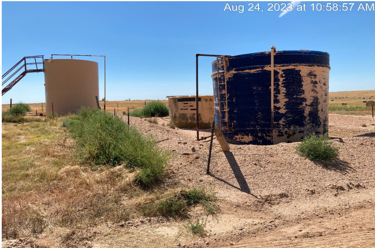
Photo 5. Facing southeast toward the tanks. Fencing is inadequate around the tanks.
