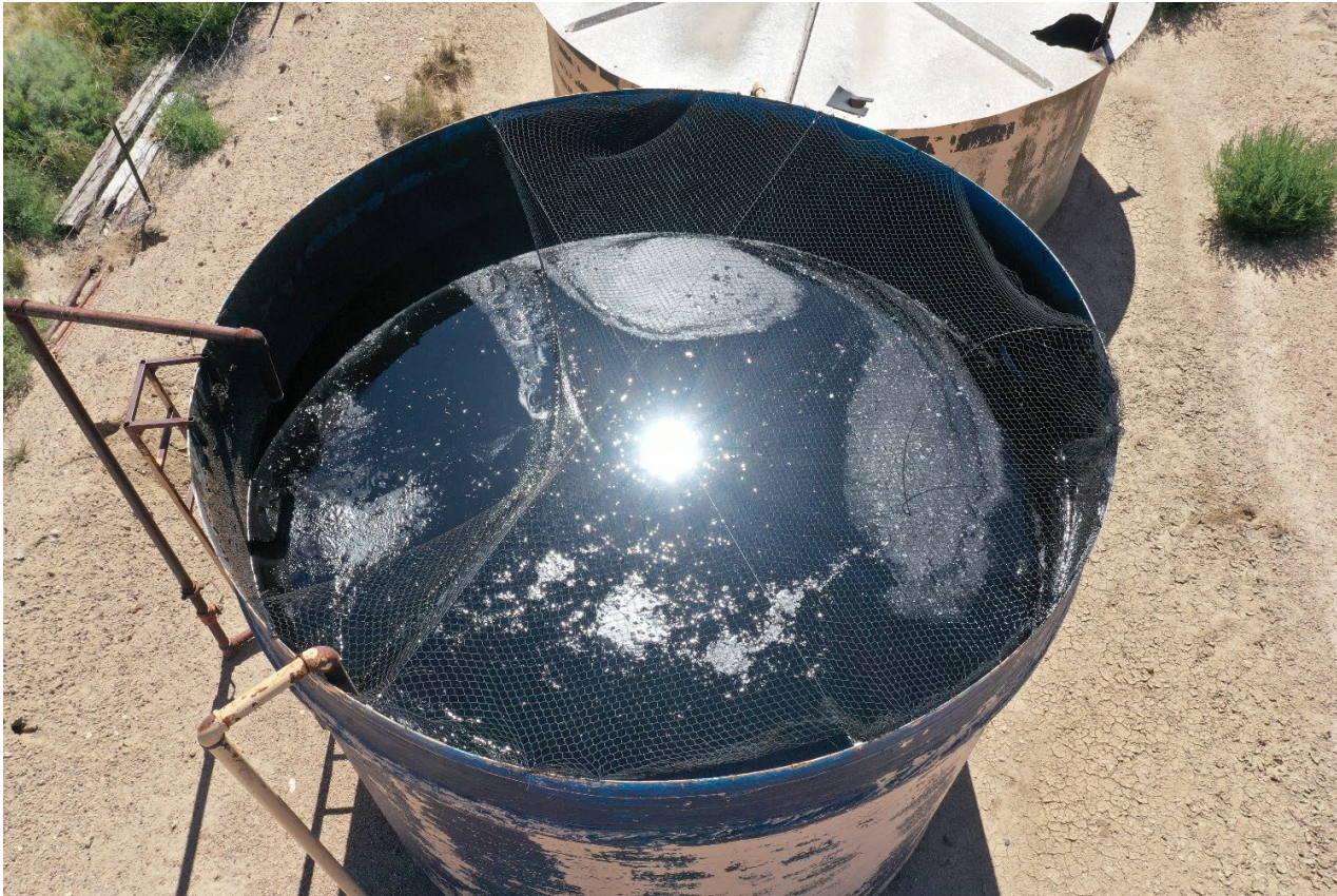
Photo 6. The netting on the open top tank needs to be repaired to prevent wildlife entry.
