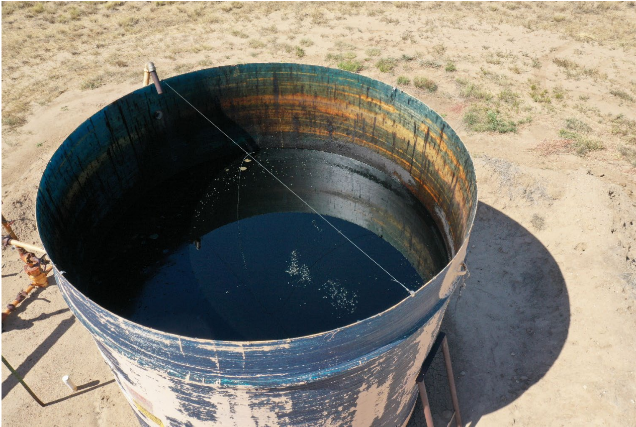
Photo 7. Drone photo looking down at the open top tanks shows no netting over the tank. Tank is approximately \frac{3}{4} full of crude oil. Previous corrective action was not completed.
