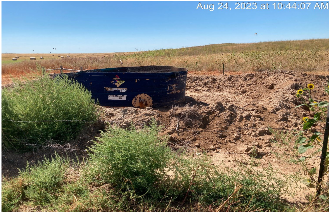
Photo 2. The berm around the tank has been built up however soils were not compacted to be impermeable.
