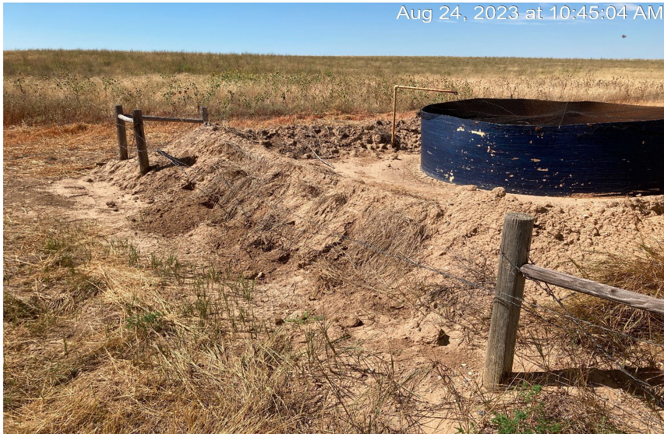
Photo 4. The fence around the open top tank is inadequate to prevent livestock entry and is not maintained. Previous corrective action was not completed.
