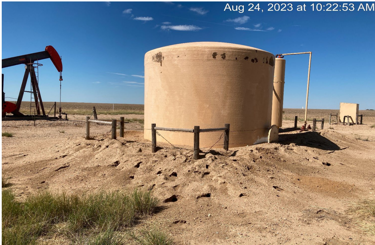
Photo 5. Facing toward the tank. The berm around the tank is inadequate to contain a spill.
