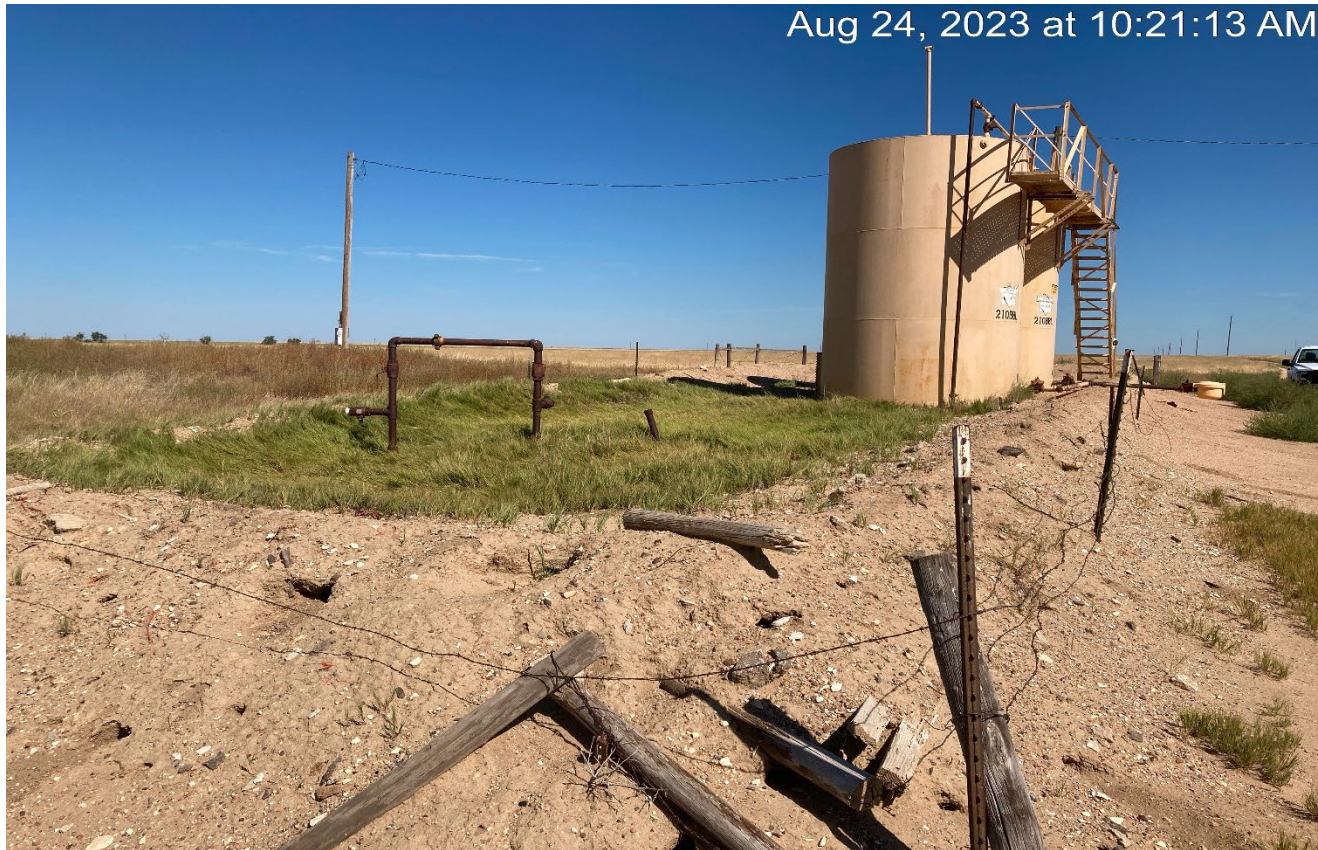
Photo 3. The fence around the tank battery is inadequate to prevent livestock entry and is not maintained.
