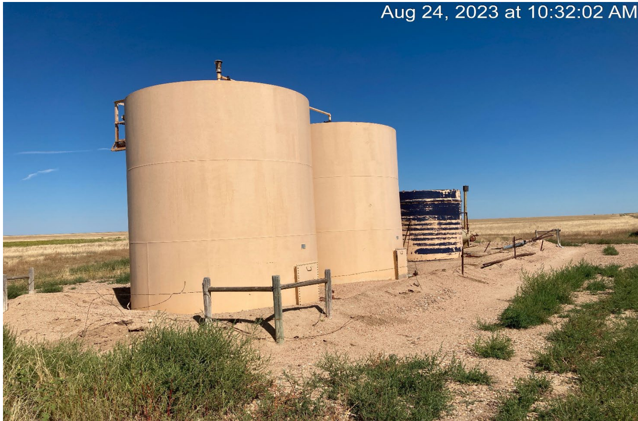
Photo 2. fence around the tank is inadequate to prevent livestock entry and is not maintained. The berm around the tank is insufficient to contain a spill (150% of tank capacity) and has animal borrows the sides.
