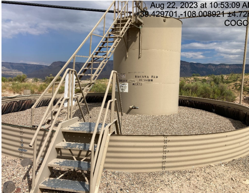
Tank battery lacking proper signage
