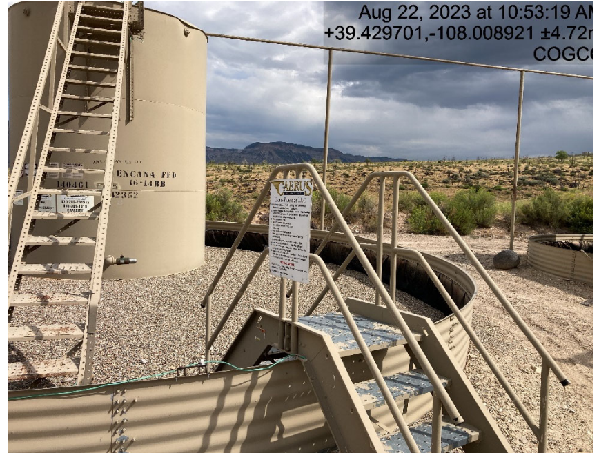
Tank battery lacking proper signage
