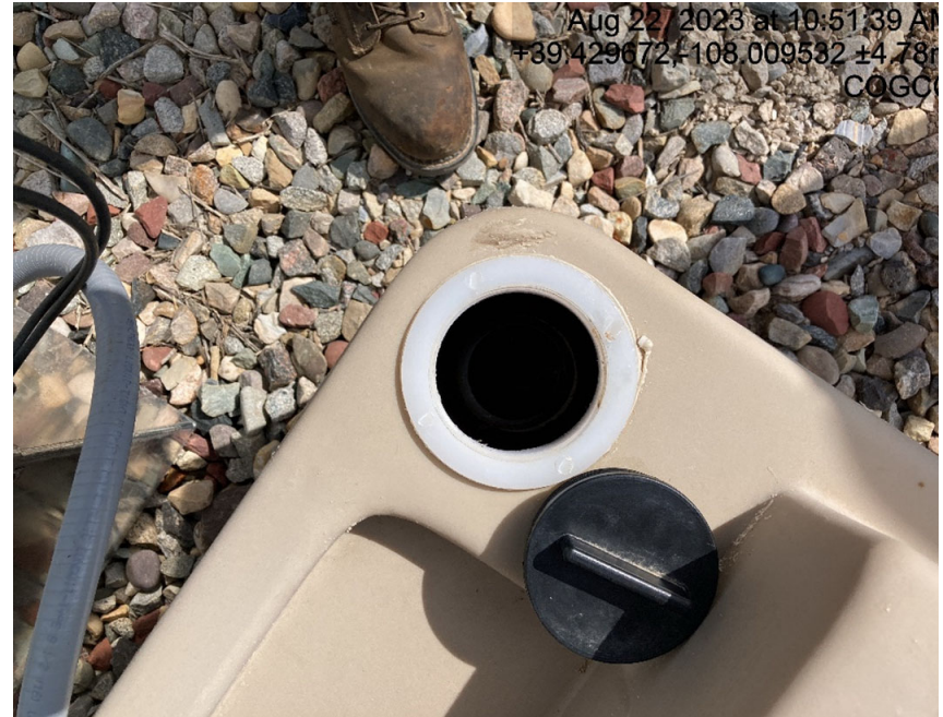
Chemical tank containment full of fluid
