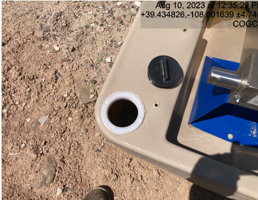
Chemical tank containment full of fluid
