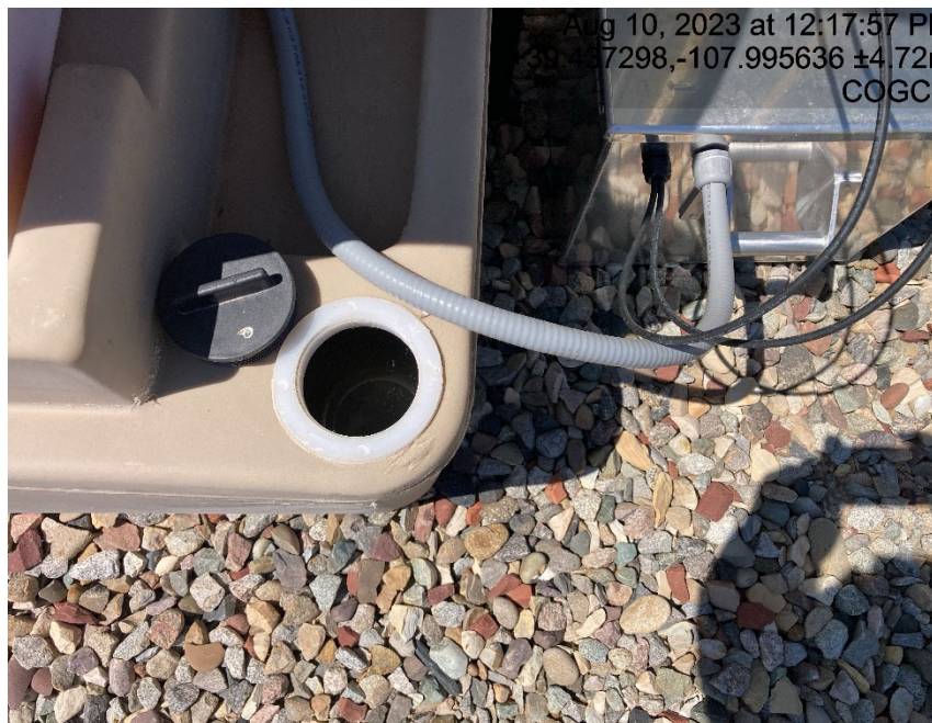
Chemical tank containment is full of fluid
