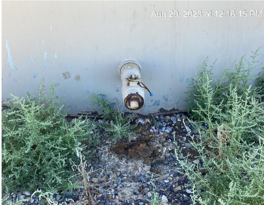
Leak. Stained soil
