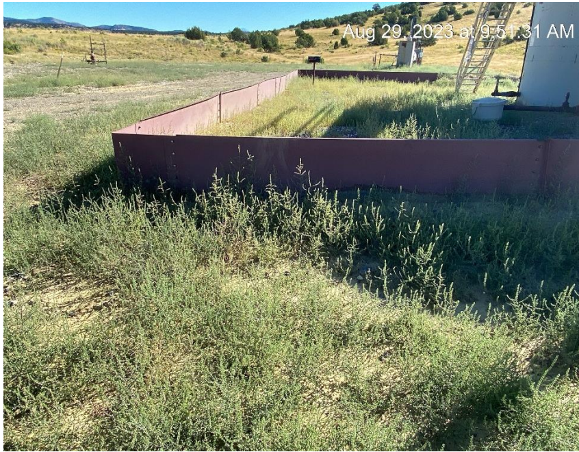
Location from Southwest corner
