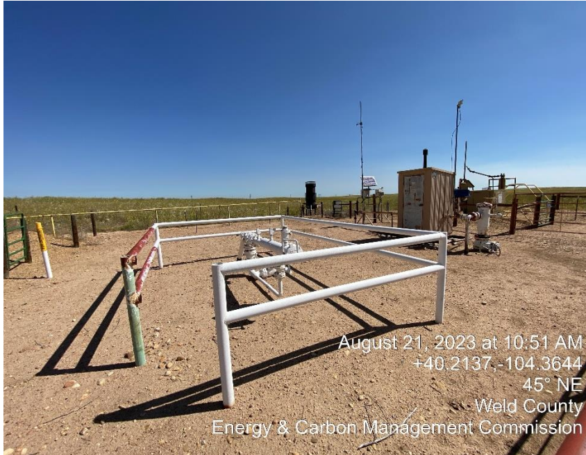
Pig Station & Gas Meter Run
