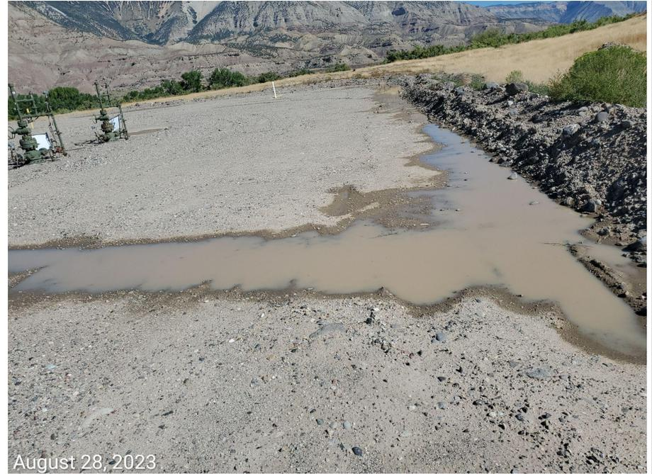
**Photo 2:** Photo shows Operator has removed the drain from the working pad perimeter; unclear if BMPs on Location area adequate to allow stormwater discharge.
