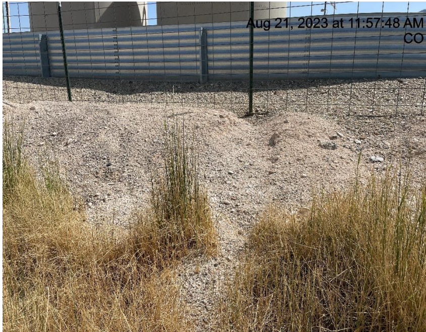
Photo # 6942 Erosion of berm & transport of sediment off location & into a vegetated area
