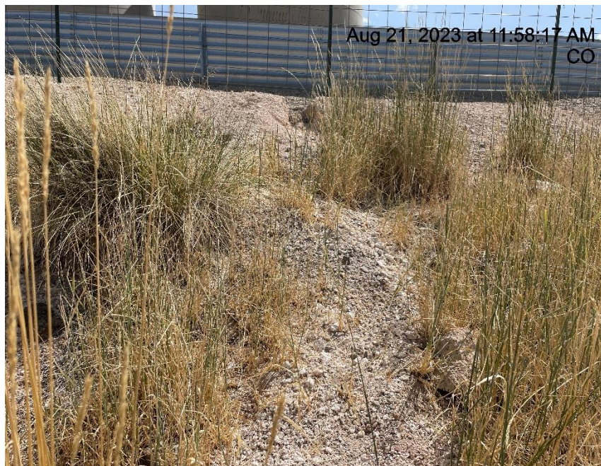
Photo # 6945 Erosion of berm & transport of sediment off location & into a vegetated area
