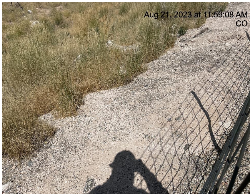
Photo # 6947 Erosion of berm & transport of sediment off location & into a vegetated area
