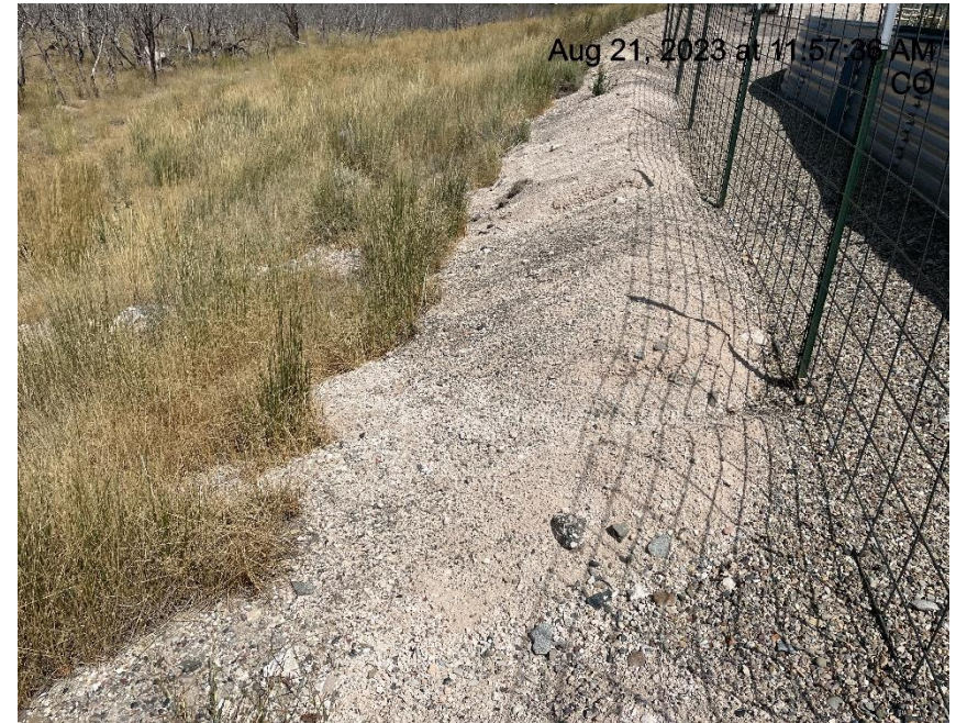
Photo # 6942 Erosion of berm & transport of sediment off location & into a vegetated area
