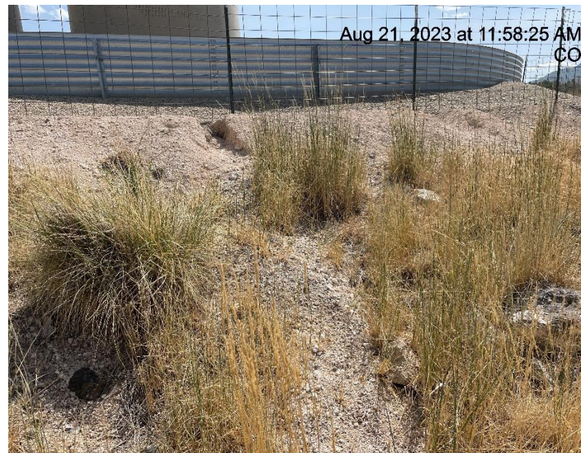
Photo # 6946 Erosion of berm & transport of sediment off location & into a vegetated area
