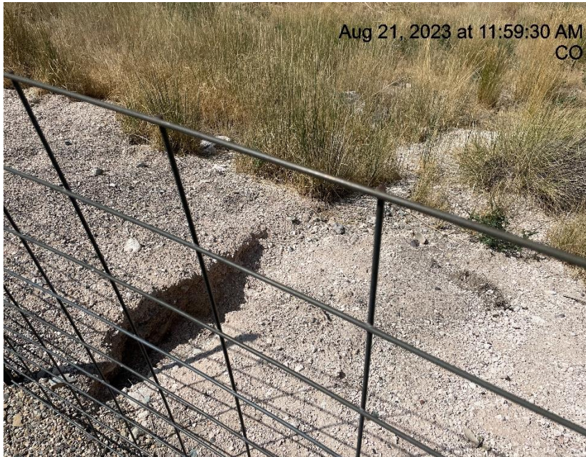
Photo # 6949 Erosion of berm & transport of sediment off location & into a vegetated area
