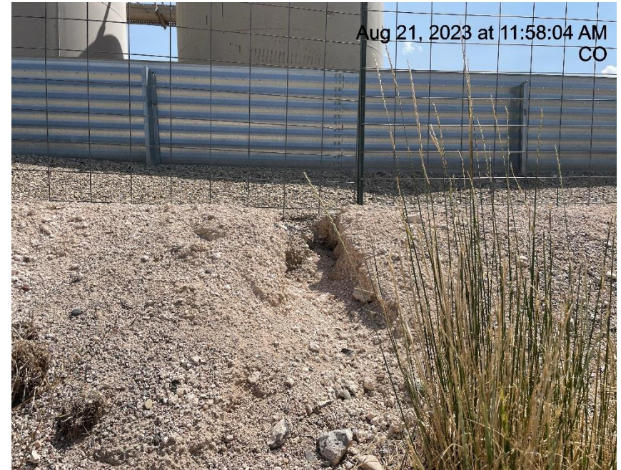
Photo # 6944 Erosion of berm & transport of sediment off location & into a vegetated area
