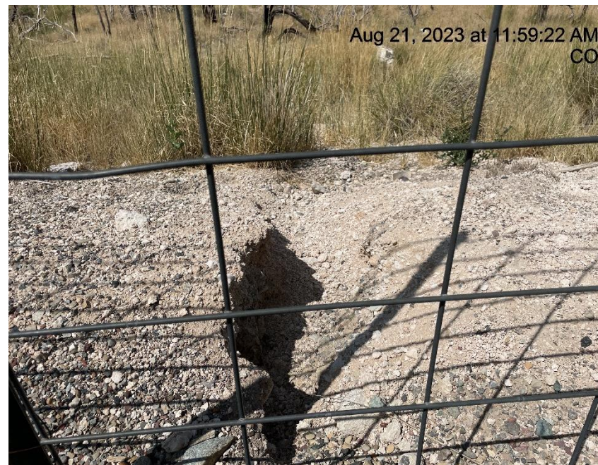
Photo # 6948 Erosion of berm & transport of sediment off location & into a vegetated area
