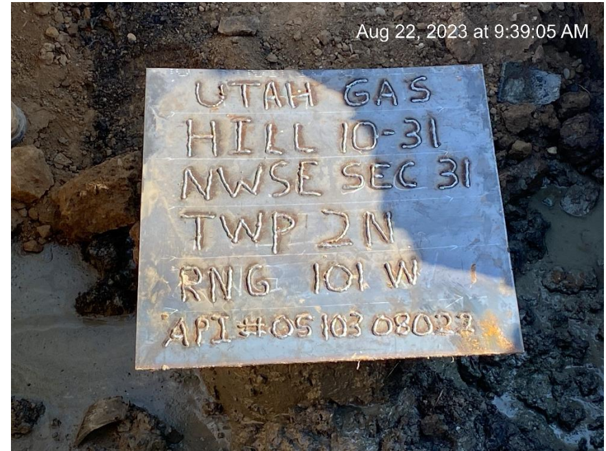
Below ground PA marker. Tack welded to Surface casing.
