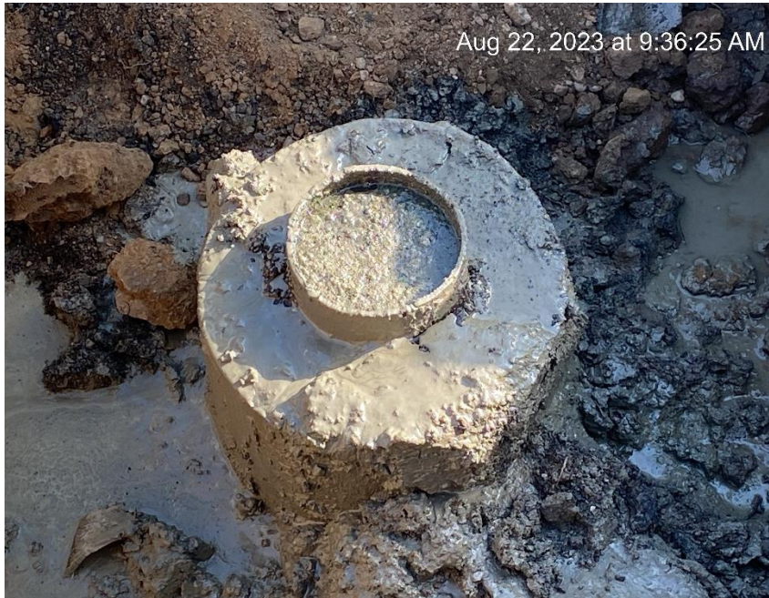
Conductor and Surface casing before PA marker.
