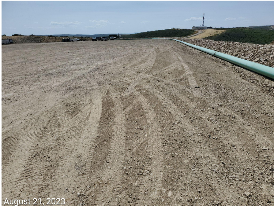
Photo 9: Slope drains along perimeter of the WPS not implemented per SWMP.
