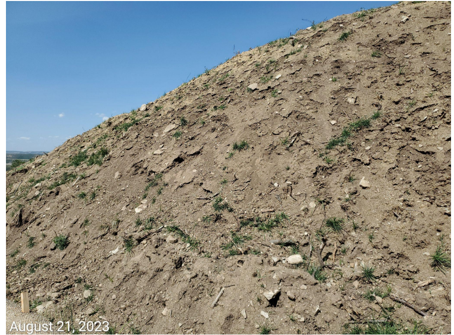
Photo 7: Photos examples showing hydromulch at the topsoil stockpiles is in disrepair.
