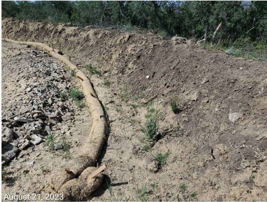
Photo 7: Photos examples showing hydromulch at the topsoil stockpiles is in disrepair.
