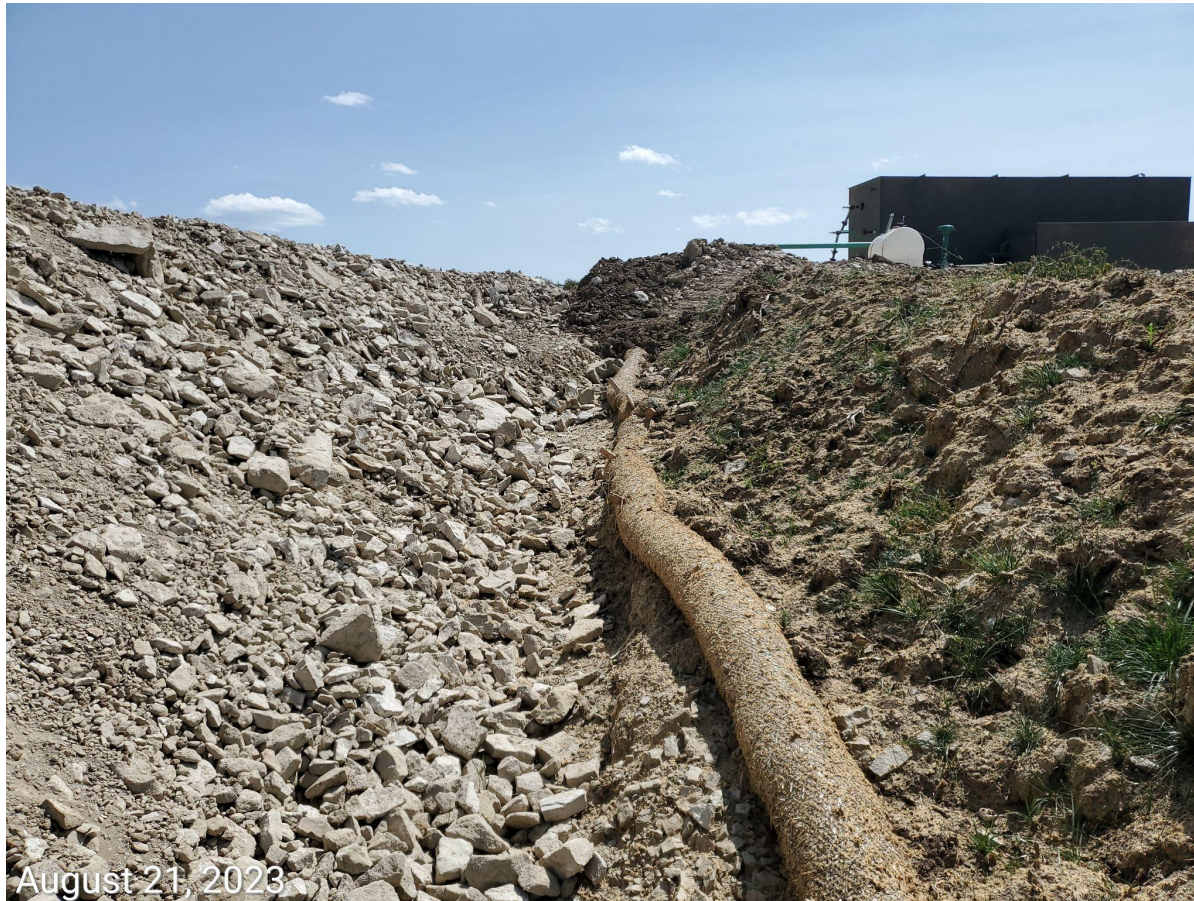
Photo 4: Sediment trap and culvert on the south end of the Location not installed. Ditch on SE end not installed.
