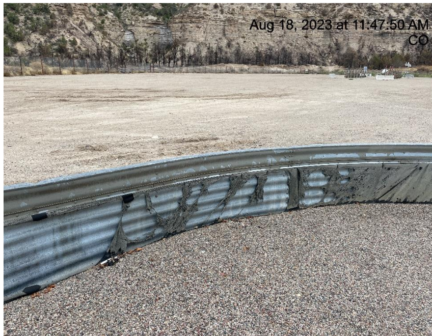
Photo # 6522 Liner needs maintenance
