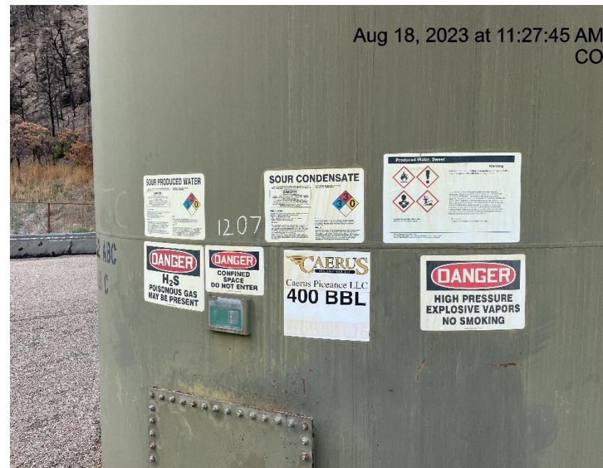
Photo # 6476 Tank/label missing required information
