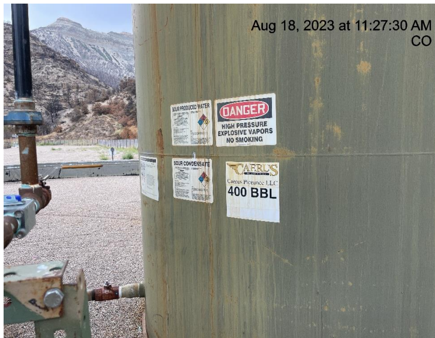
Photo # 6475 Tank/label missing required information
