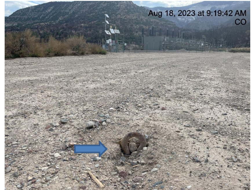
Photo # 6238 Same unmarked deadman from a different angle
