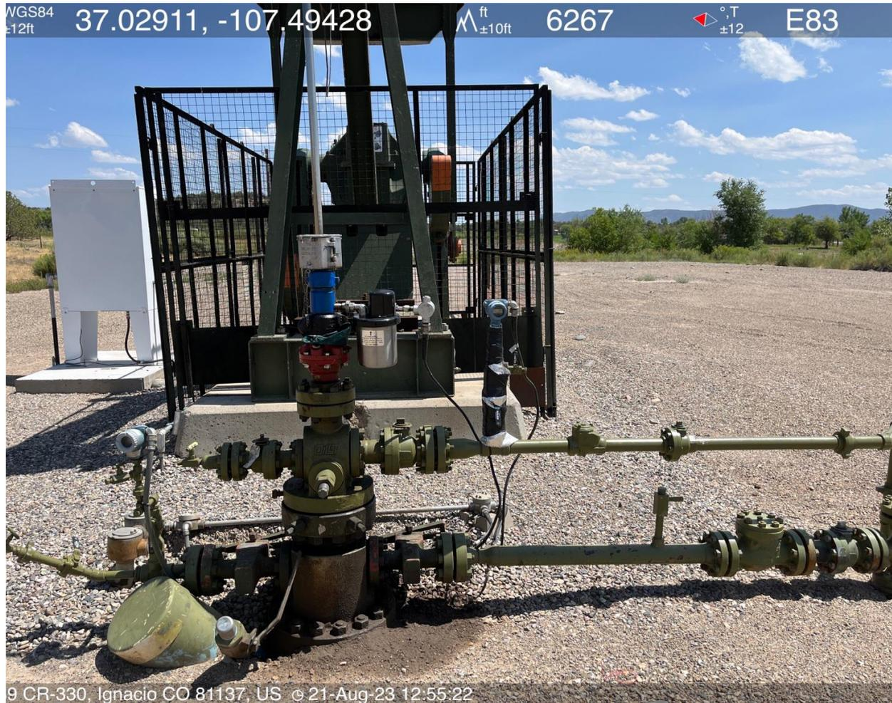
Photo #2 View of the wellhead assembly.
