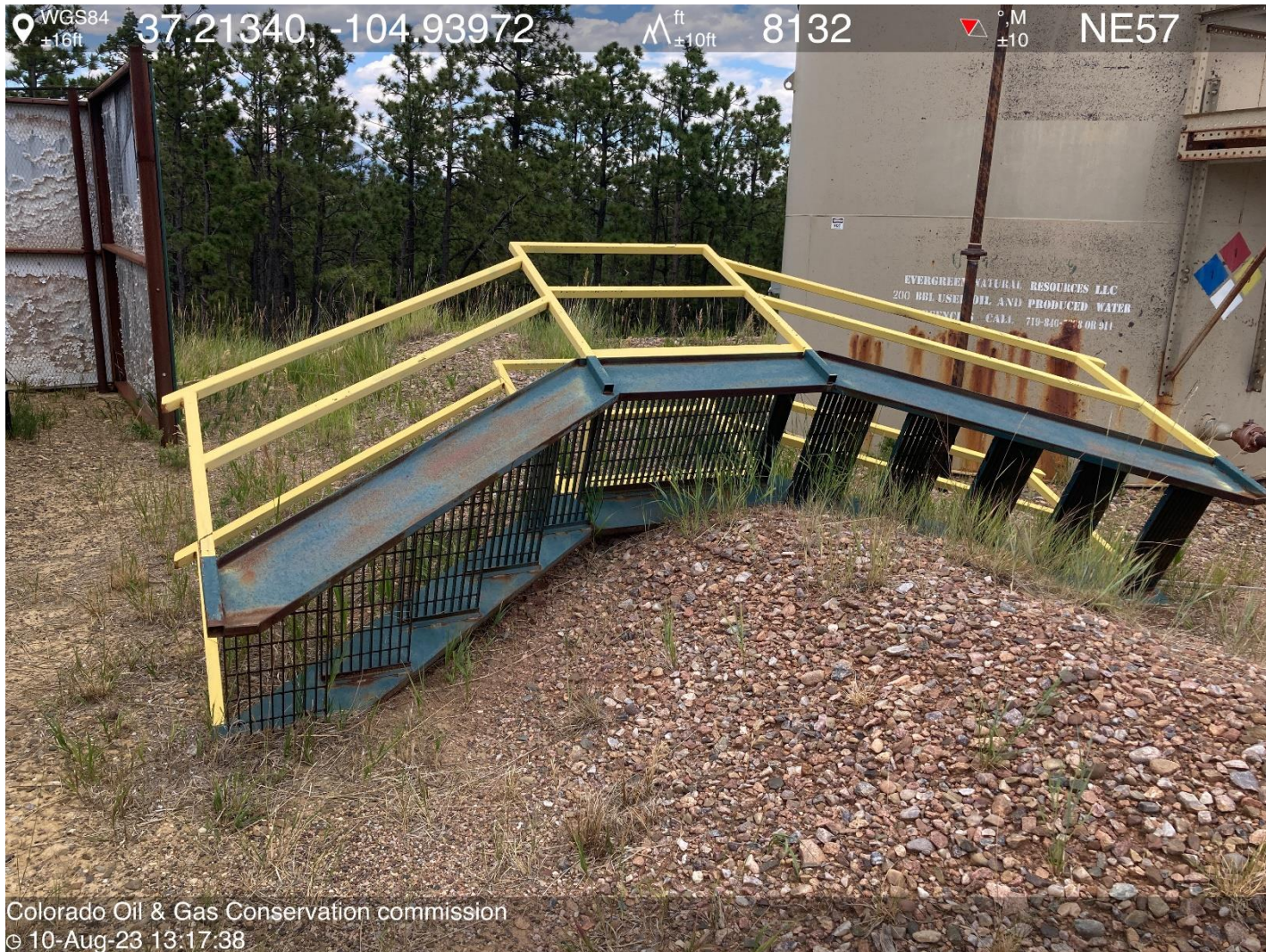
PHOTO 5: UNUSED EQUIPMENT STORED ON LOCATION (SET OF STAIRS LYING ON ITS SIDE OVER TANK BATTERY BERMS). REMOVE OR USE UNUSED EQUIPMENT PER RULE 606. CA DATE 9-21-2023.
