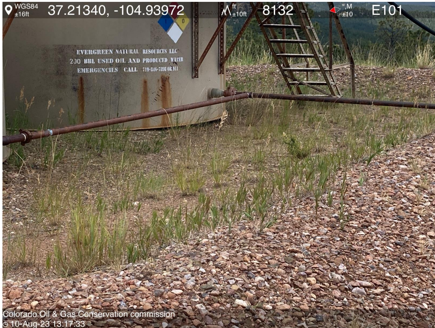
PHOTO 6: WEEDS INSIDE TANK BATTERY BERMS. REMOVE ALL VEGETATION OR AND INSIDE TANK BATTERY BERMS PER RULE 606. CA DATE 9-21-2023.
