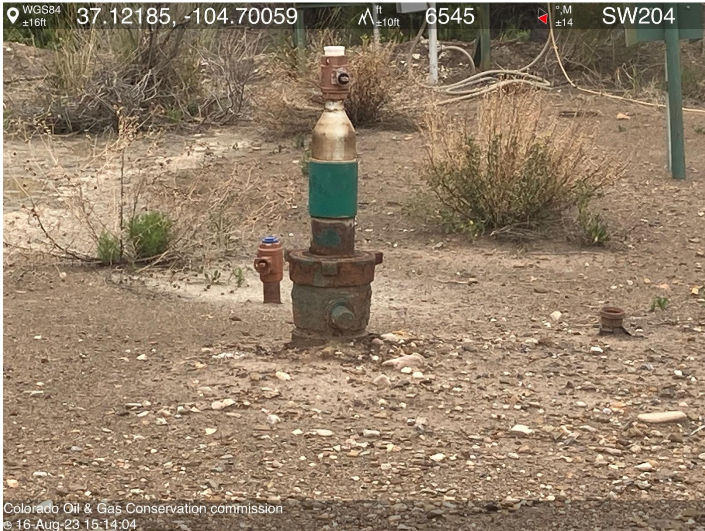
PHOTO 4: UNUSED EQUIPMENT (TWO-2" RISERS NEAR THE WELLHEAD). REMOVE OR MARK UNUSED RISERS PER RULE 606. CA DATE 9-16-2023.
