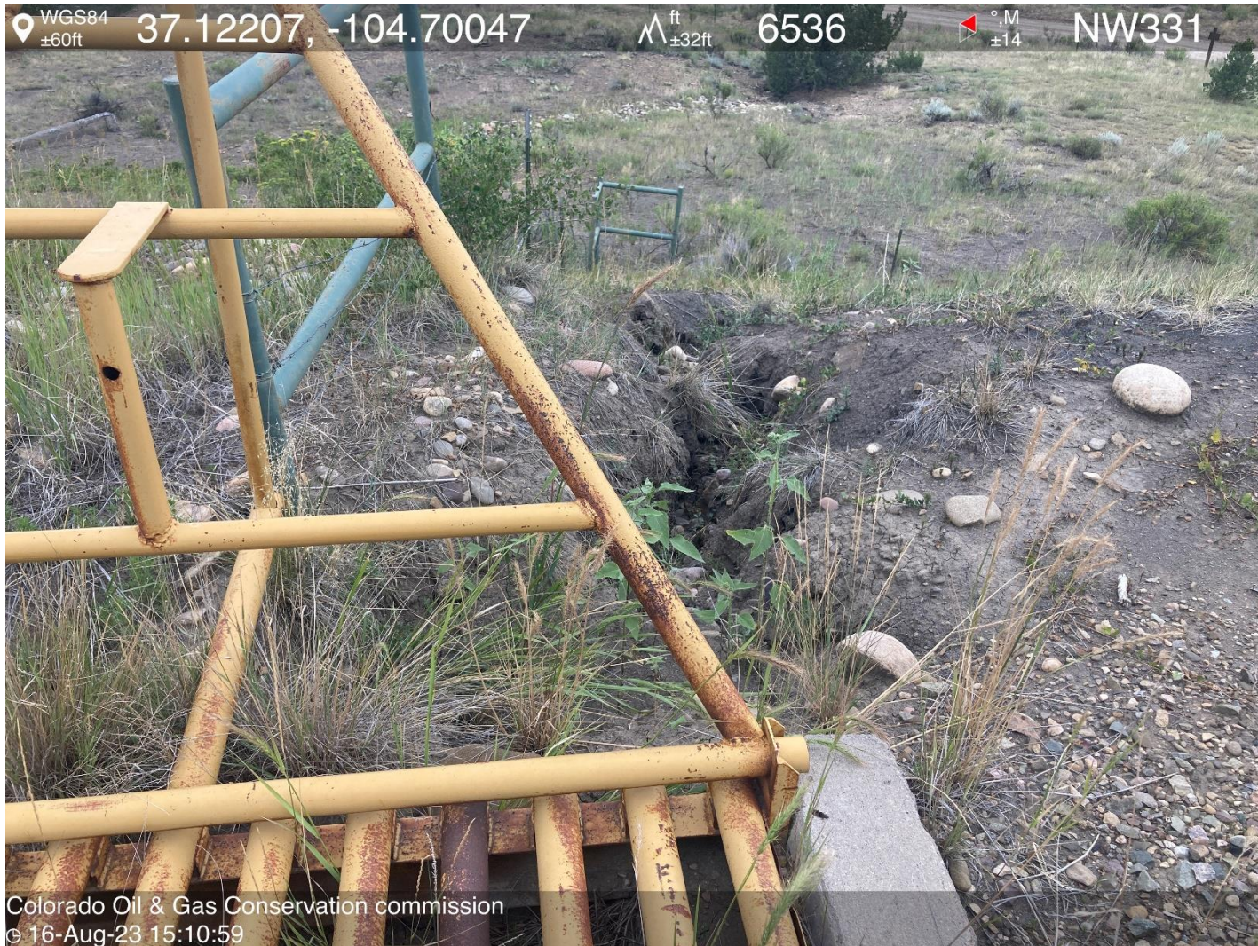
PHOTO 6: STORM WATER MANAGEMENT IS INADEQUATE ON DOWN SLOPE SIDE OF CATTLE GUARD AT ENTRANCE OF LOCATION. INSTALL STORM WATER MANAGEMENT BMP'S PER RULE 1002. CA DATE 9-16-2023.
