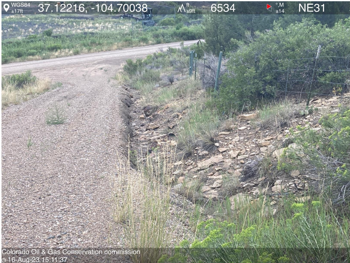
PHOTO 7: STORMWATER HAS ERODED THE DITCH ON EAST SIDE OF ROW. INSTALL OR MAINTAIN STORM WATER MANAGEMENT BMP'S PER RULE 1002. CA DATE 9-16-2023.
