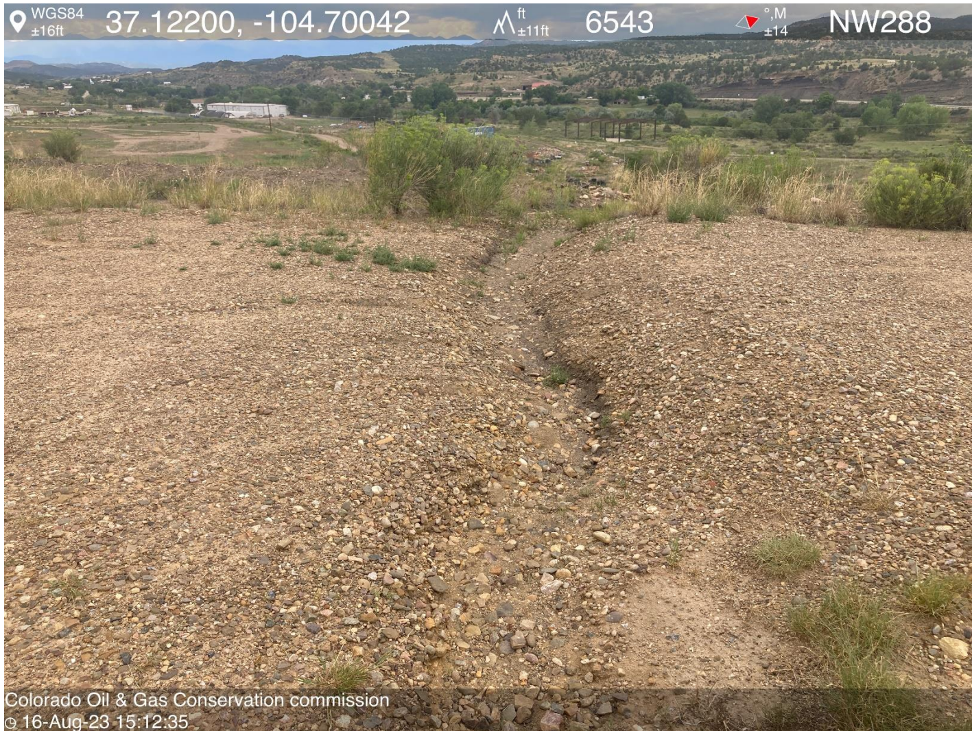
PHOTO 6: STORM WATER MANAGEMENT IS INADEQUATE AT ENTRANCE OF LOCATION, THERE IS A DITCH THAT IS WASHING OUT AND MAKING IT DIFFICULT FOR VEHICLES TO ENTER LOCATION. INSTALL OR MAINTAIN STORM WATER MANAGEMENT BMP'S PER RULE 1002. CA DATE 9-16-2023.
