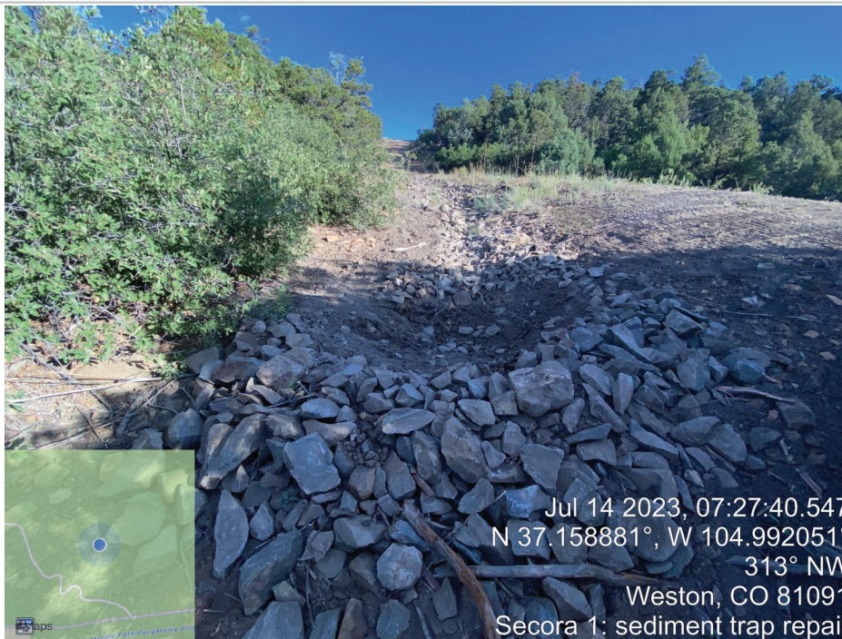
Photo Point 5: Sediment Trap Repair
