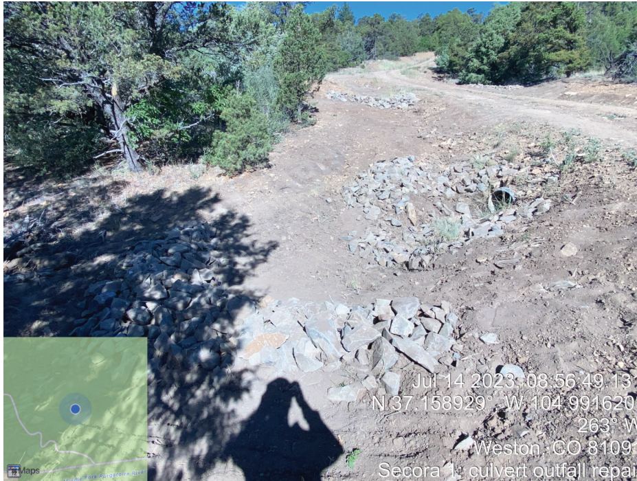
Photo Point 8: Check Dam Repair, Culvert Outfall Maintenance
