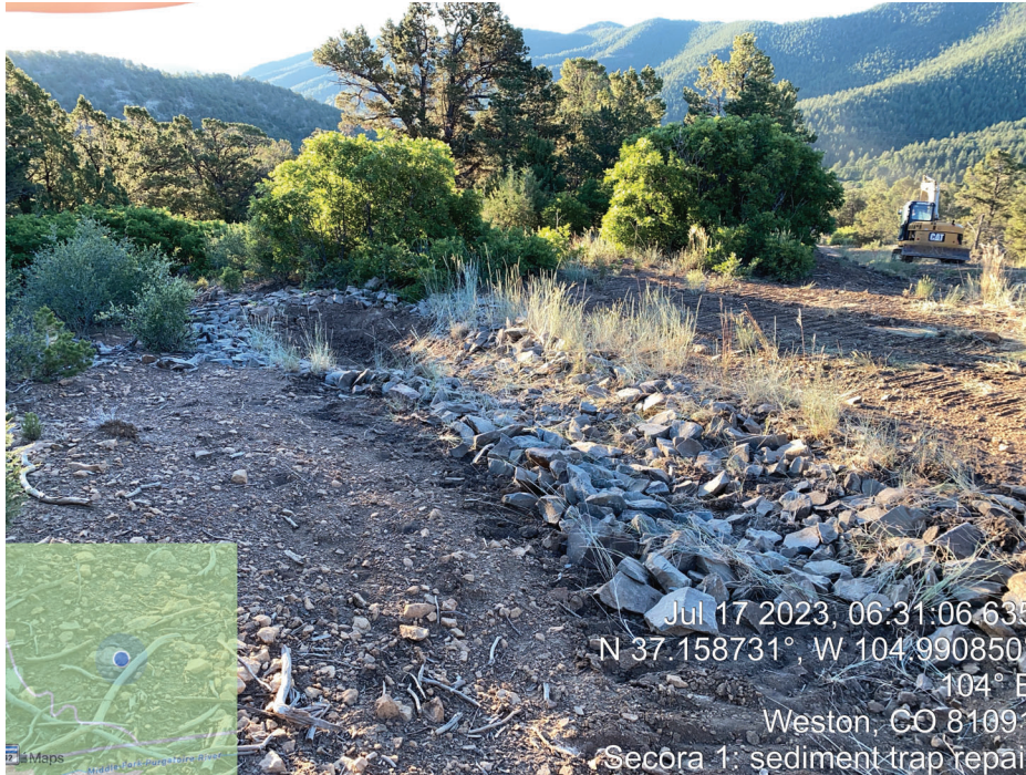
Photo Point 15: Check Dam Repair
