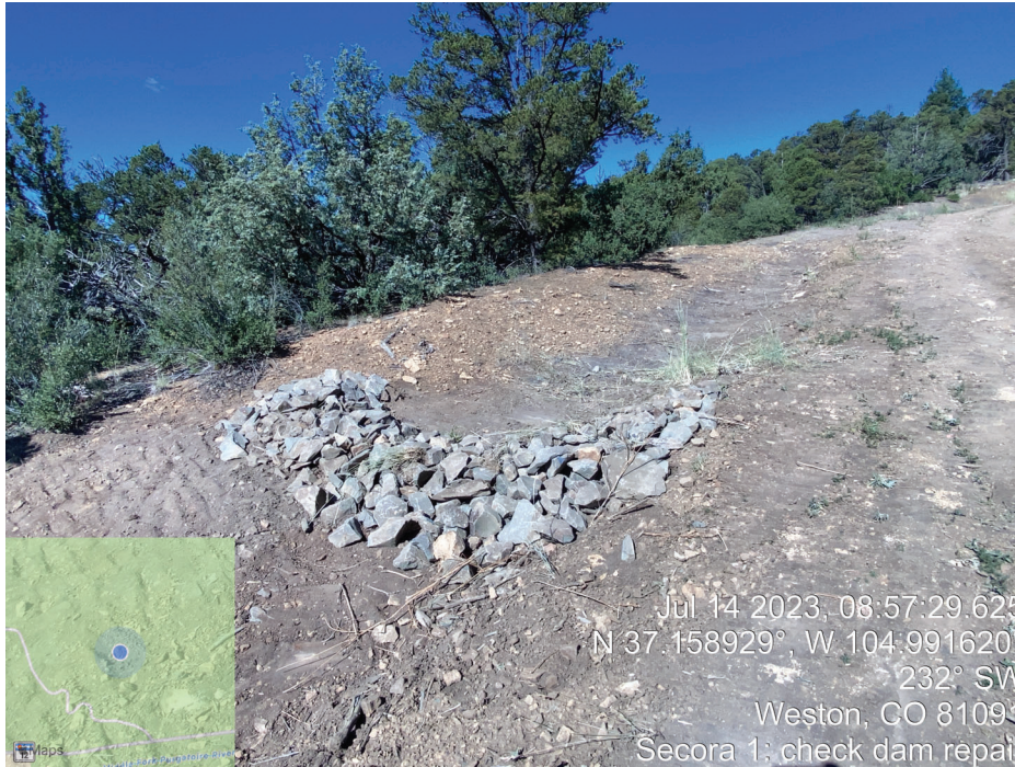
Photo Point 11: Check Dam Repair
