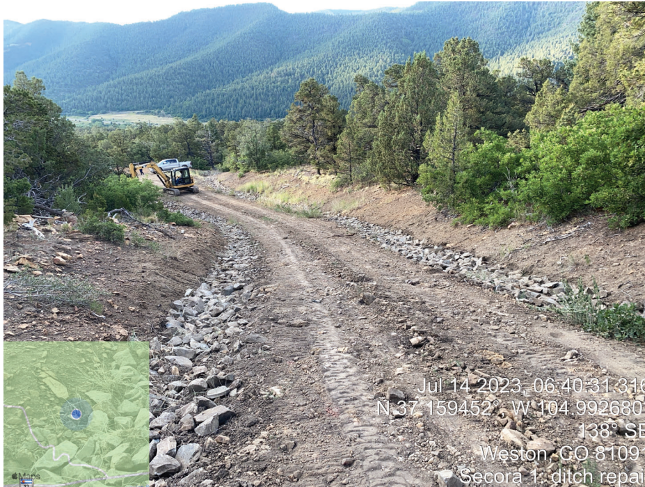
Photo Point 3: Armored Ditch Repair
