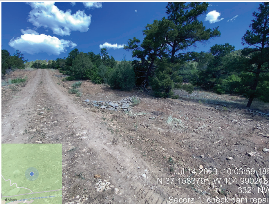
Photo Point 19: Check Dam Repair
