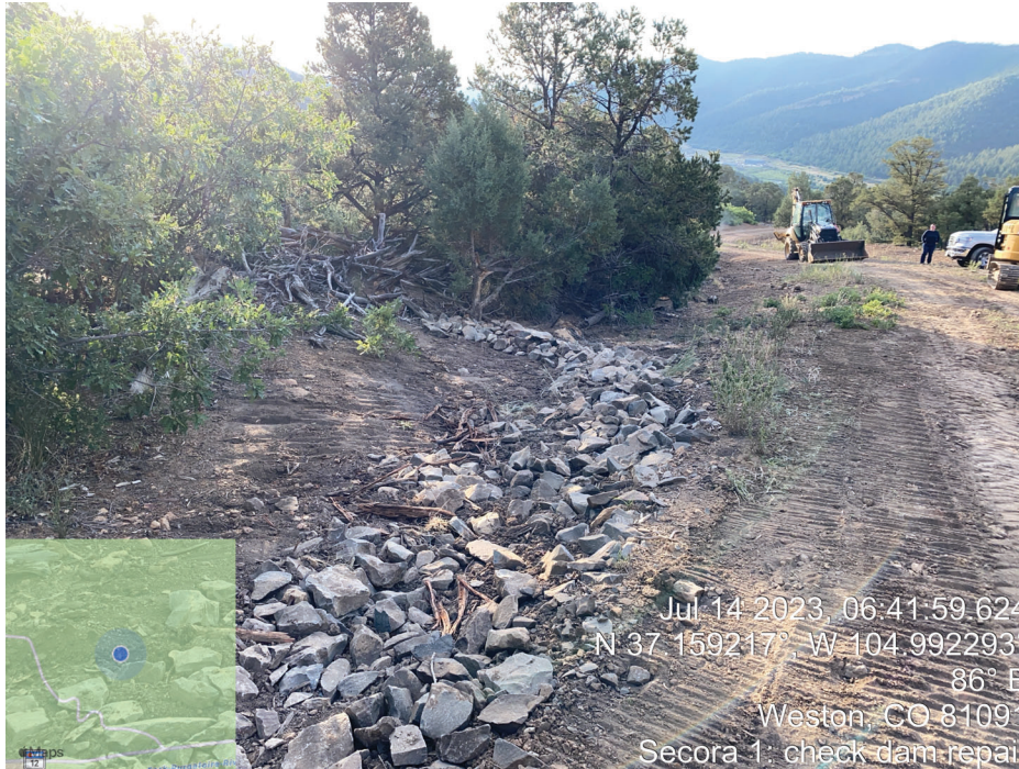
Photo Point 5: Sediment Trap Repair
