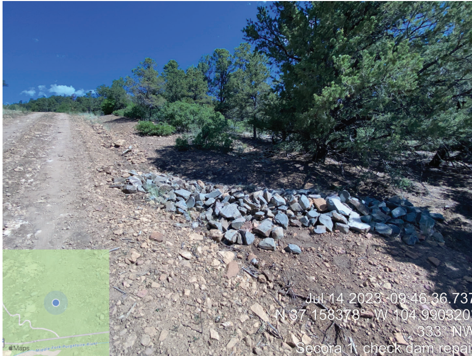
Photo Point 19: Check Dam Repair
