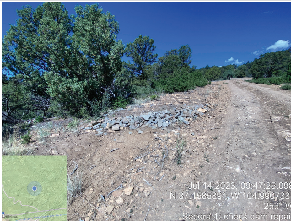
Photo Point 15: Check Dam Repair
