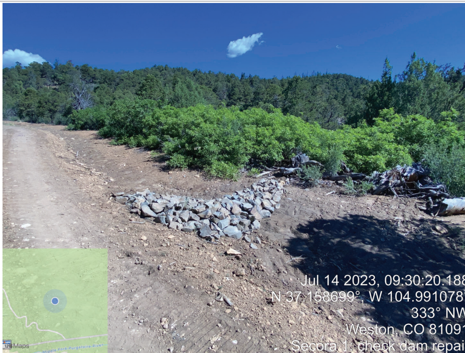
Photo Point 13: Check Dam Repair
