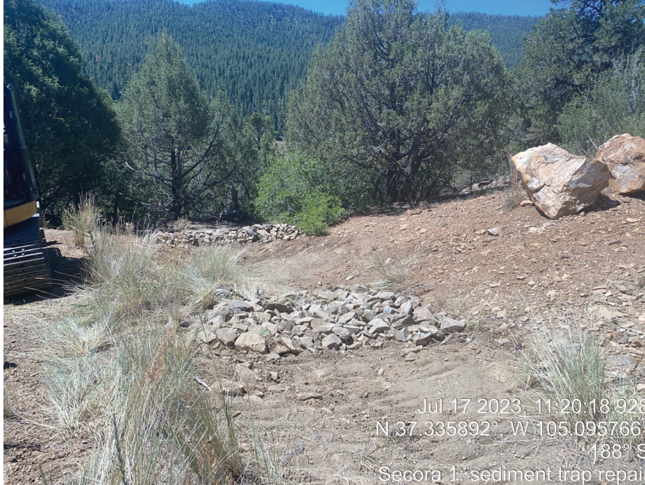
Photo Point 30: Sediment Trap Repair
