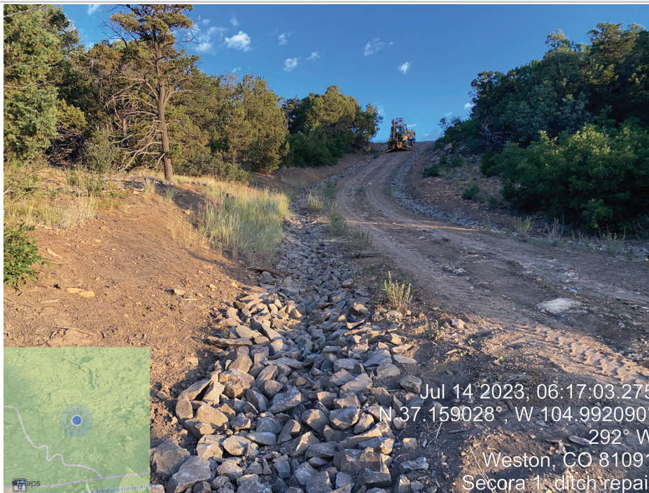
Photo Point 3: Armored Ditch Repair
