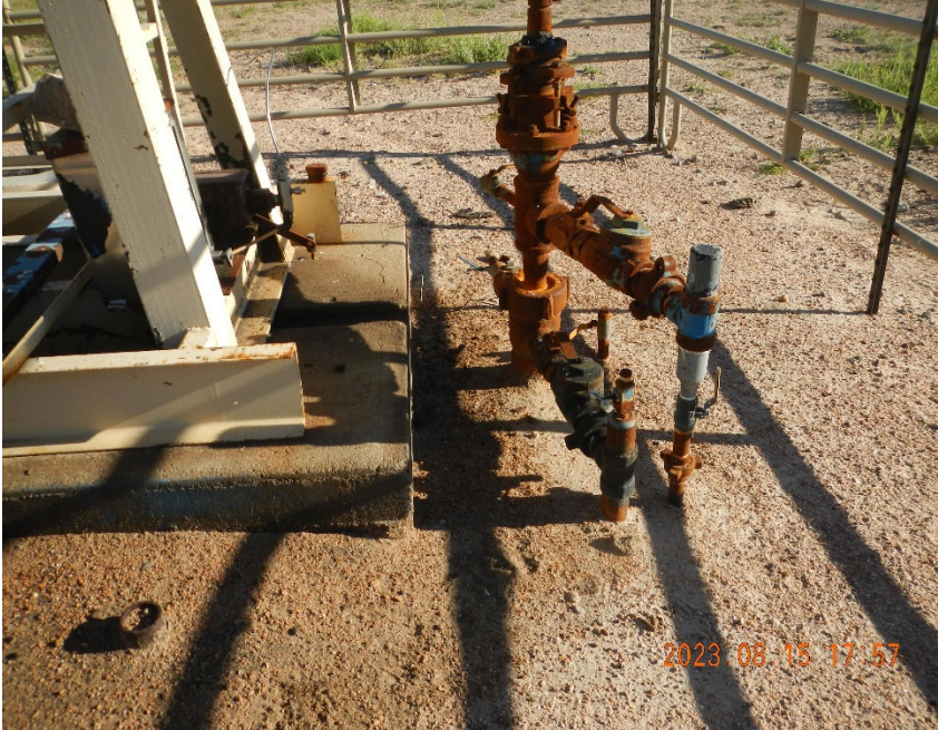
3. Additional view of stained soils around wellhead and pumping unit.
