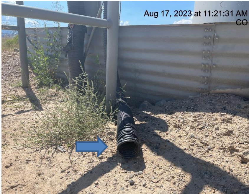
Photo # 6151 Flowline heating insulation open ended
