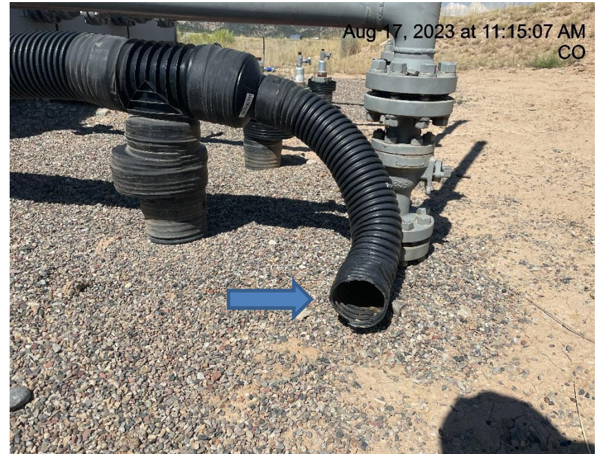
Photo # 6142 Flowline heating insulation open ended
