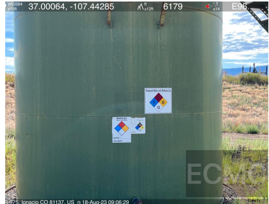
Photo #4. View of no tank volume labeling. Corrective action not completed.
