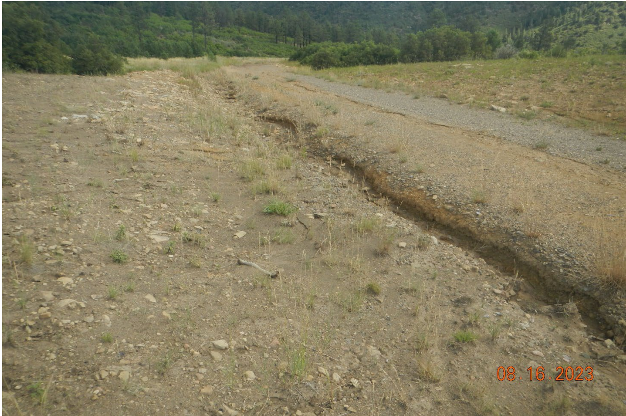
Photo 2. Facing north toward the access road at the location. There is erosion along the road side at the location.
