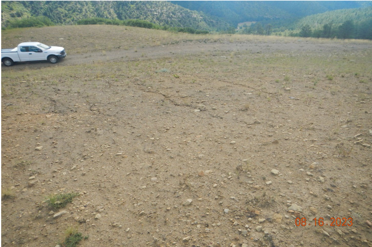
Photo 4. Facing east at the location. This portion of the location is not stabilized with vegetation cover and has signs of erosion.
