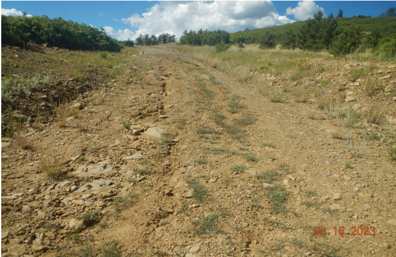
Photo 1. Facing southeast along the access road near the location. There is erosion along this area of the road that needs to be repaired and stabilized.
