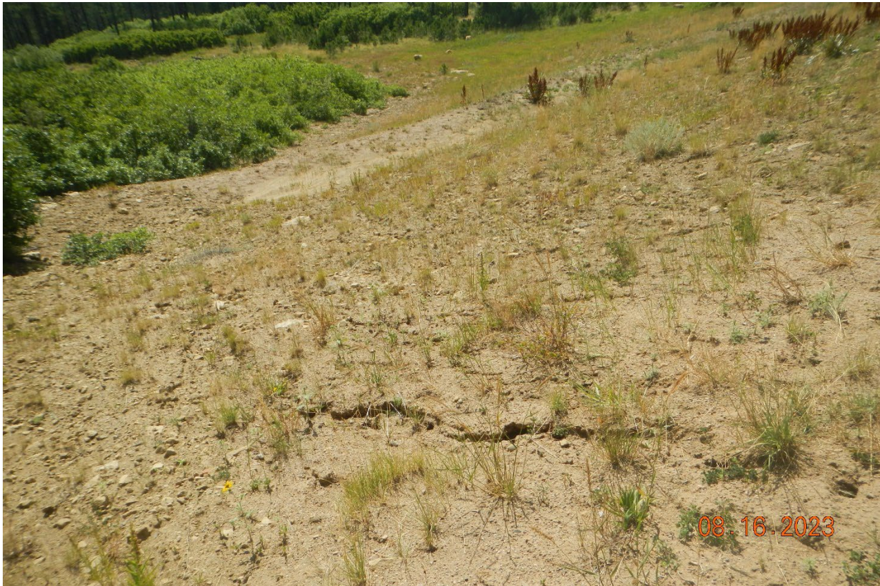
Photo 10. Facing southeast down the bottom of the location. This portion of the location is not stabilized with vegetation cover and has signs of erosion.
