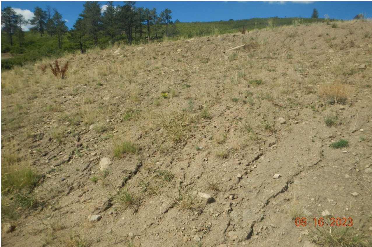
Photo 9. Southeast side of the location facing west. This portion of the location is not stabilized with vegetation cover and has signs of erosion.
