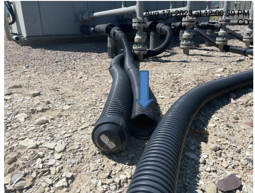
Photo # 6183 Flowline heating insulation open ended.
