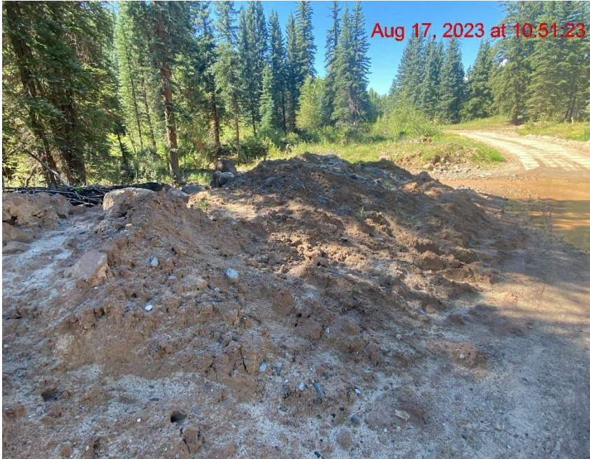
Unprotected Soil Stockpiles Near Clear Fork Crossing – Photo #05921
