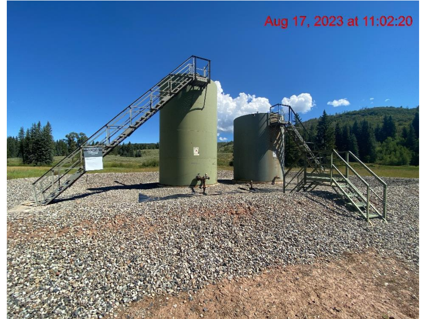
Tank Battery – Photo #05930
