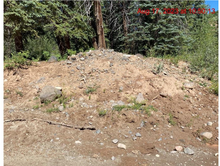
Unprotected Soil Stockpiles at Clear Fork Crossing – Photo #05920
