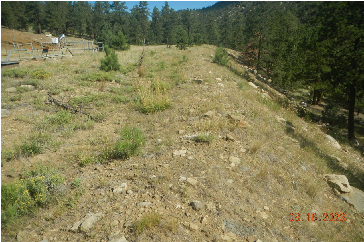
Photo 5. Facing northwest along the fill slope which is stabilized with perennial vegetation.
