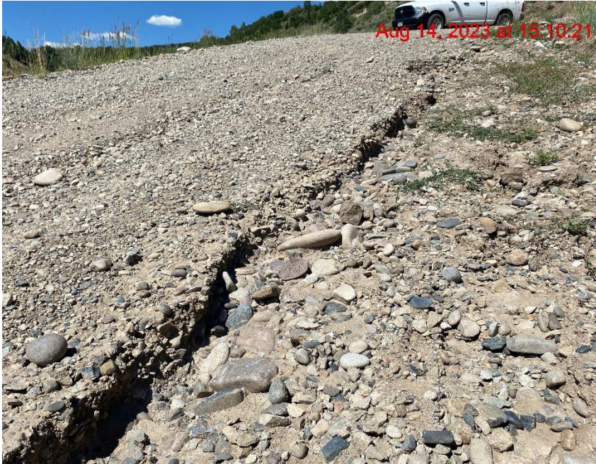
Rill Erosion Cutting Through Lease Road – Photo #05872
