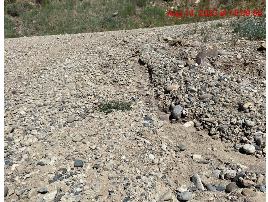
Rill Erosion Cutting Through Lease Road – Photo #05871
