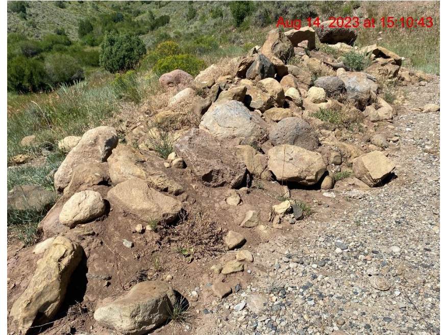
Unprotected Soil Stockpile – Photo #05873
