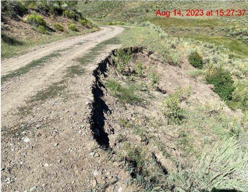
Insufficient Erosion Control/Road Washing Out – Photo #05876
