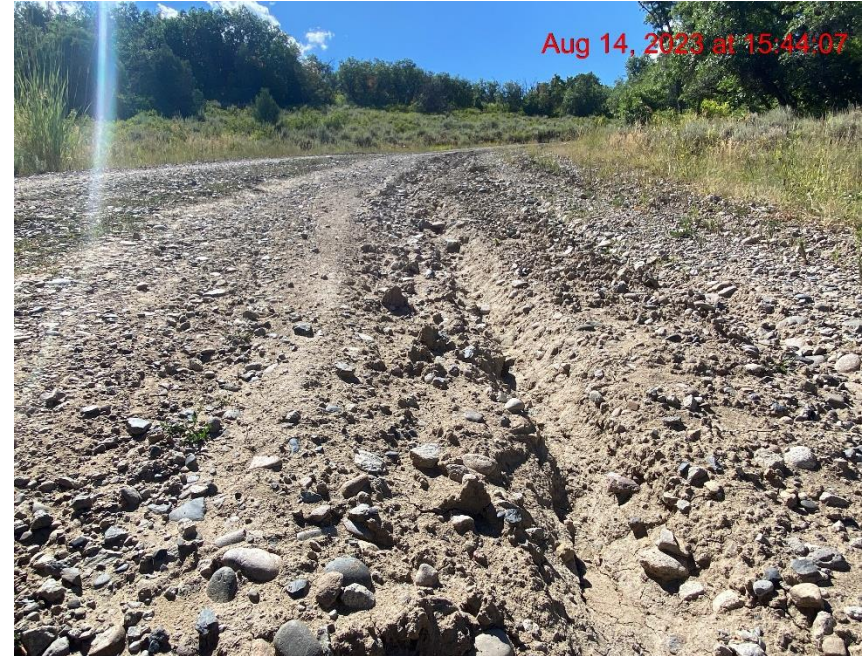
Rill Erosion Cutting Through Lease Road – Photo #05877
