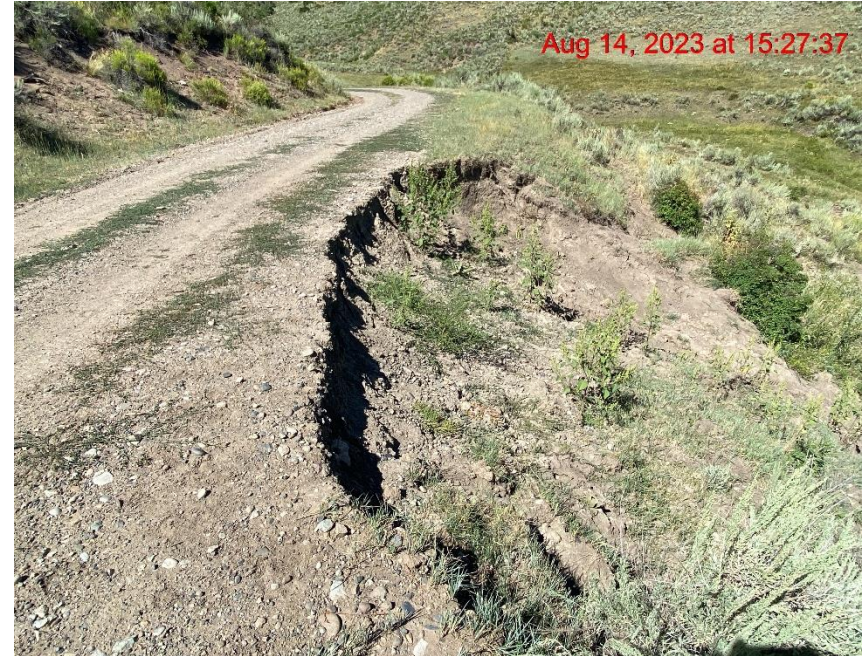
Lease Road Washing Out/Insufficient Erosion Controls – Photo #05876
