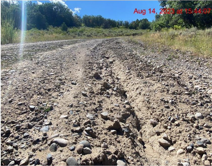
Rill Erosion on Lease Road/Insufficient Erosion Control – Photo #05877
