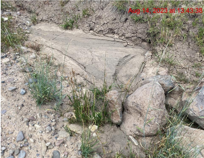
Check Dam Needs Maintenance – Photo #05839
