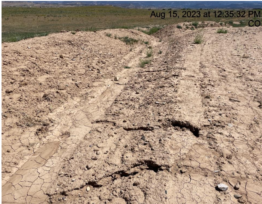
Photo # 5977 Rill erosion along ditch
