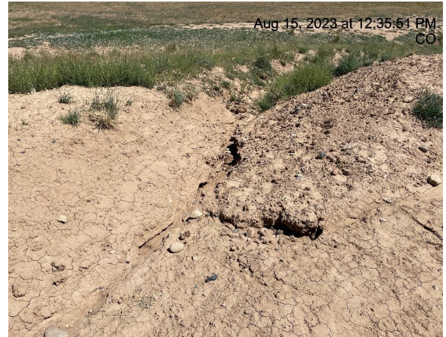
Photo # 5978 Erosion & transport of sediment/insufficient runoff controls/BMP's (NE area of location near entrance to ditch that runs off location)
