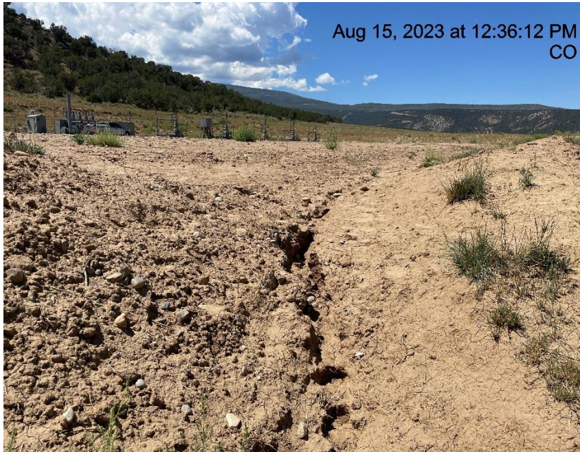
Photo # 5979 Erosion & transport of sediment/insufficient runoff controls/BMP's (NE area of location at beginning of ditch that runs off location)
