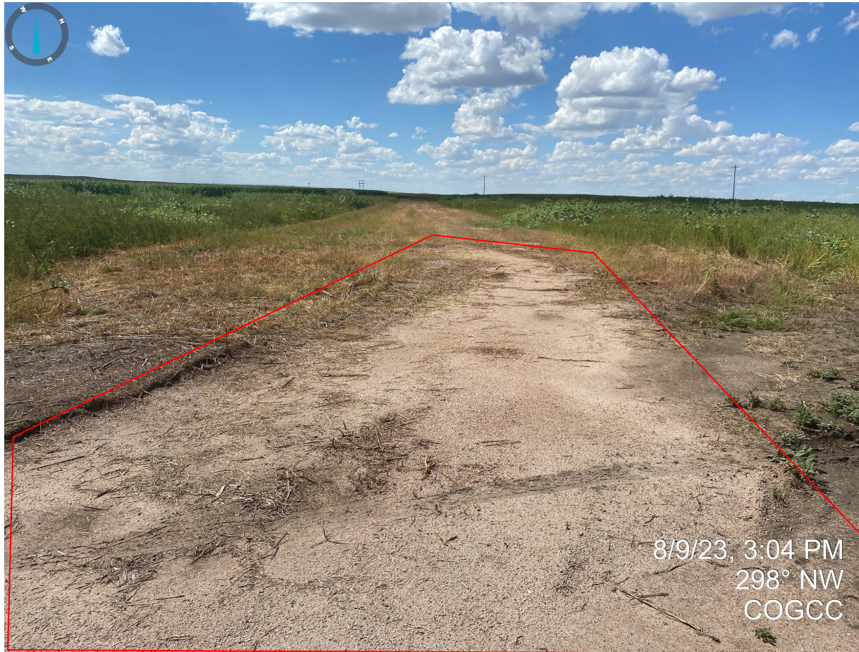
Photo 1. Road base/gravel remains on the former access road and will need to be removed per Rule 1004 regulations and standards.
