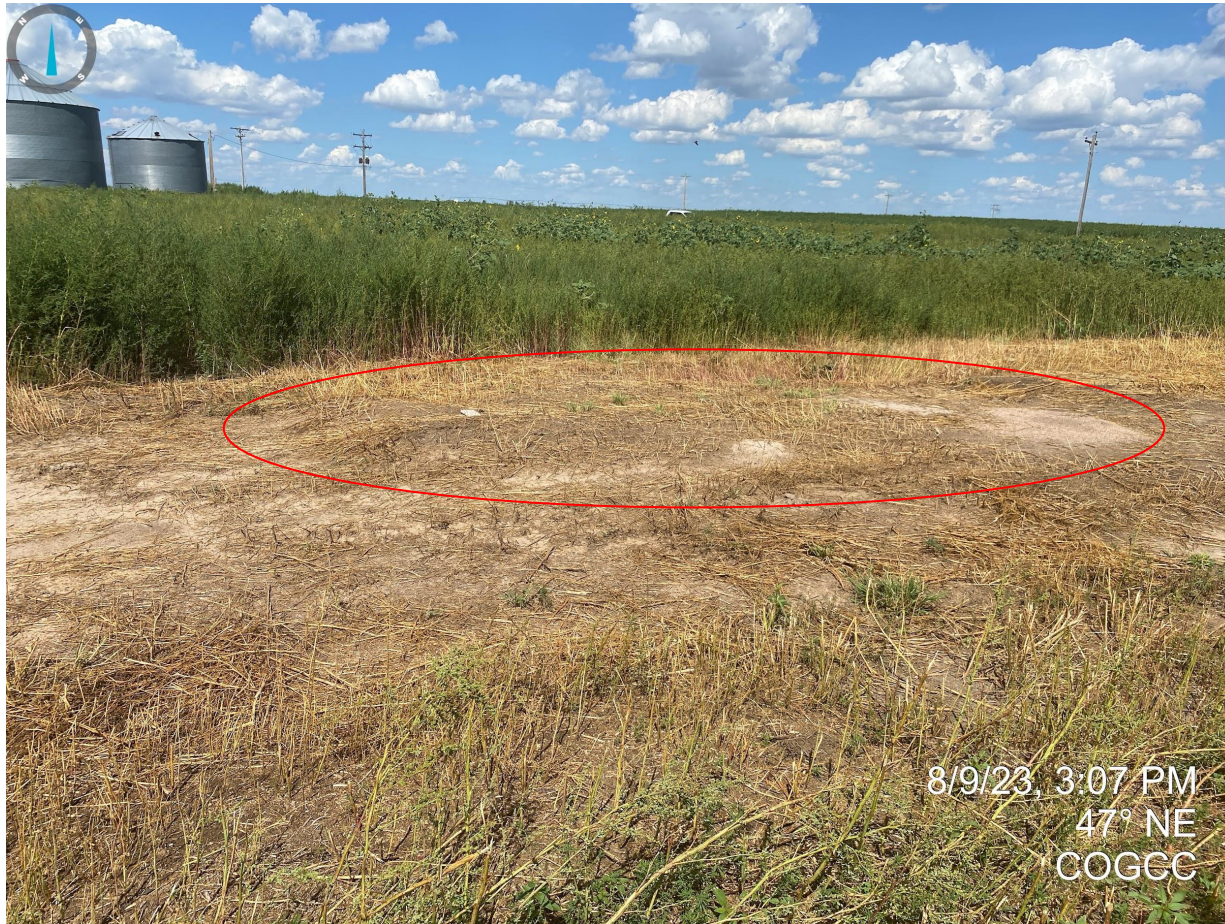
Photo 2. The former location will need to be leveled/graded as there was evidence of contouring issues at the time of this inspection (highlighted in red).
