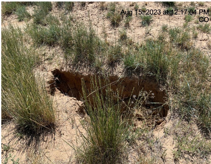
Photo # 5954 Tunnel erosion/sink hole/insufficient runoff controls/BMP's (NW corner of location near ditch)
