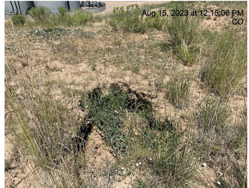
Photo # 5951 Tunnel erosion/sink hole (SW corner of location)
