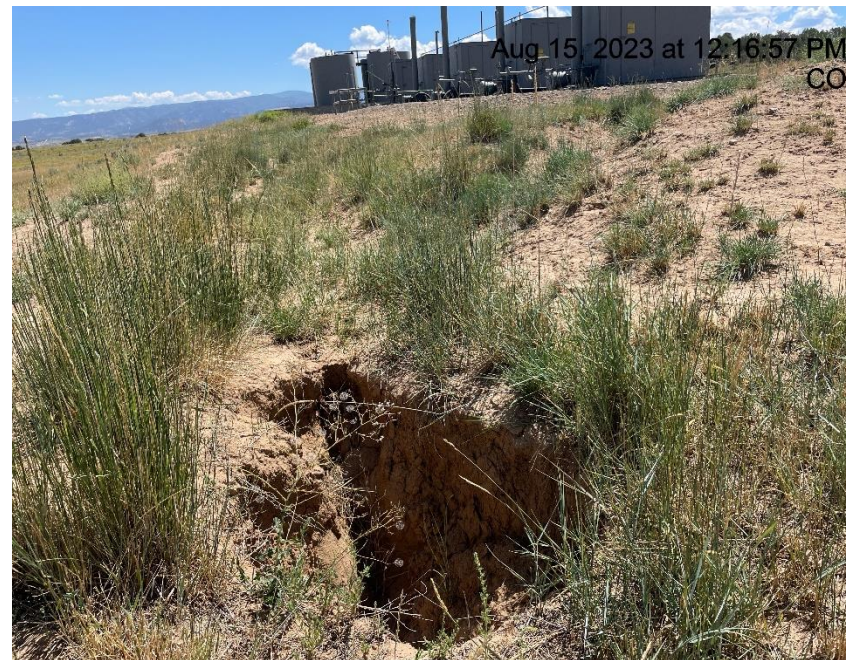
Photo # 5953 Tunnel erosion/sink hole/insufficient runoff controls/BMP's (NW corner of location in ditch)
