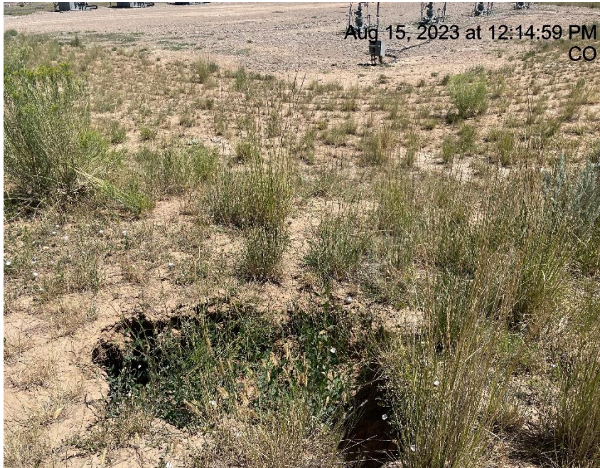
Photo # 5950 Tunnel erosion/sink hole (SW corner of location)
