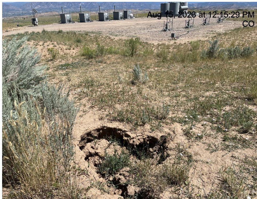
Photo # 5952 Tunnel erosion/sink hole (SW corner of location)
