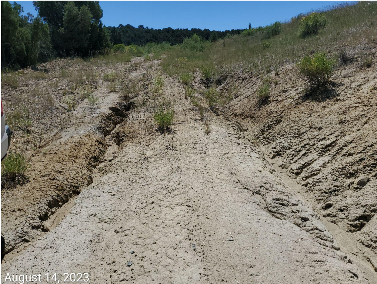
Photo 8: Photo example showing persisting erosion degradation along access road. Stormwater and erosion control measures remain inadequate. Access road has not been decompacted, recontoured, regraded and reclaimed in accordance with 1004 Rules.
