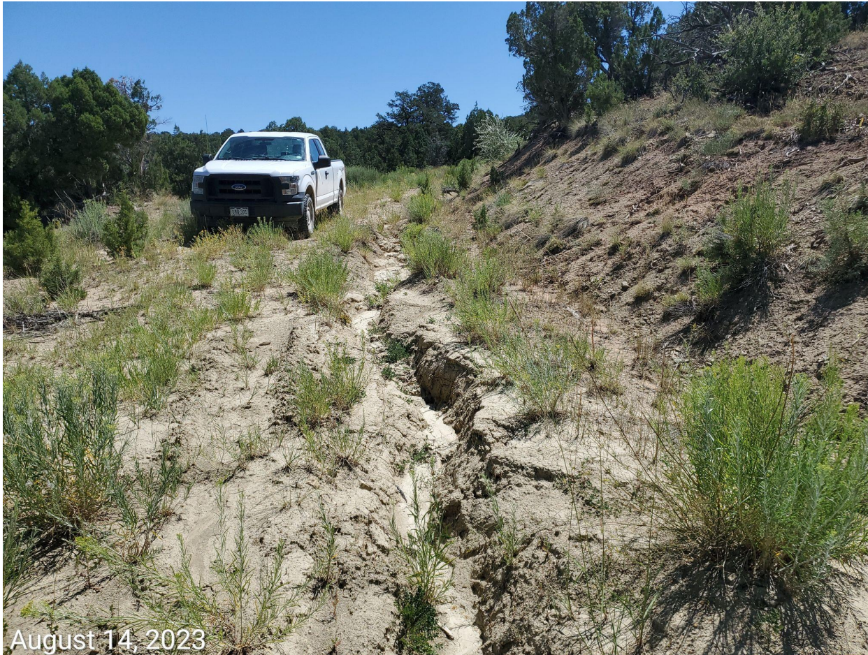
Photo 14: Photo example showing persisting erosion degradation along access road. Stormwater and erosion control measures remain inadequate. Access road has not been decompacted, recontoured, regraded and reclaimed in accordance with 1004 Rules.
