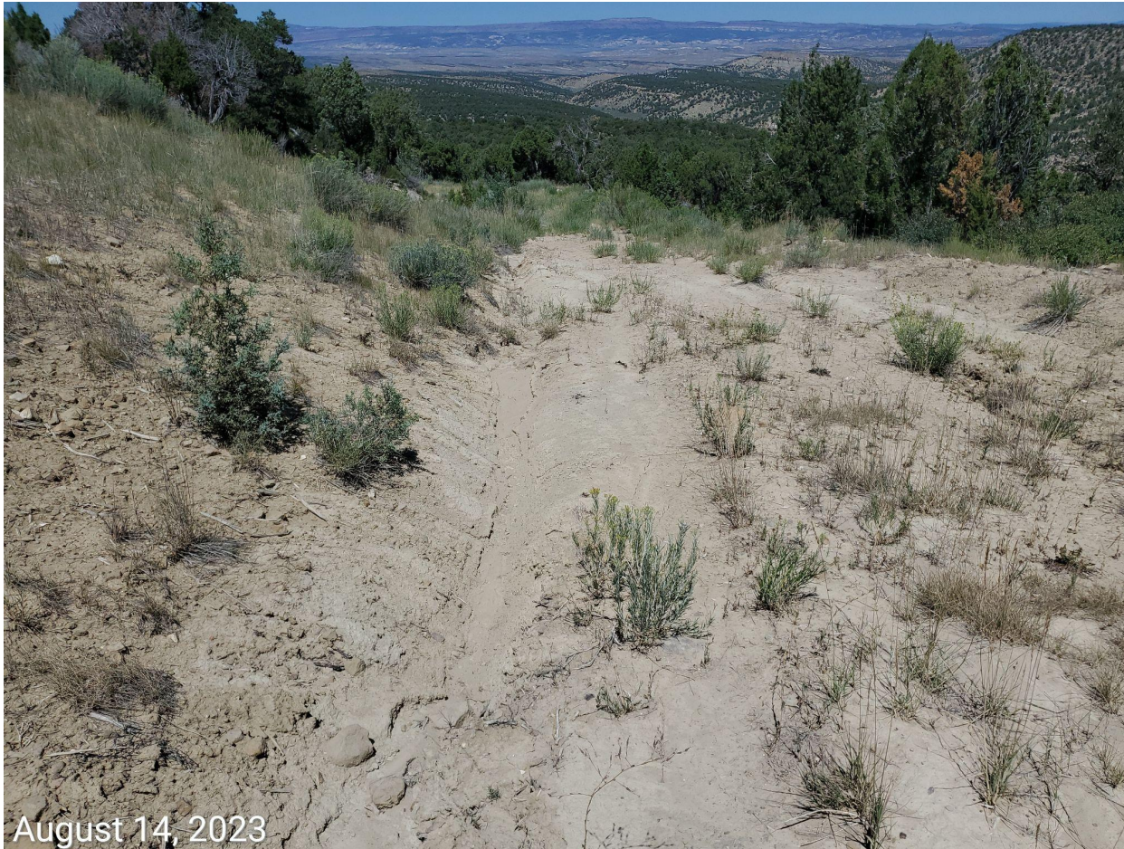
Photo 12: Photo example showing persisting erosion degradation along access road. Stormwater and erosion control measures remain inadequate. Access road has not been decompacted, recontoured, regraded and reclaimed in accordance with 1004 Rules.
