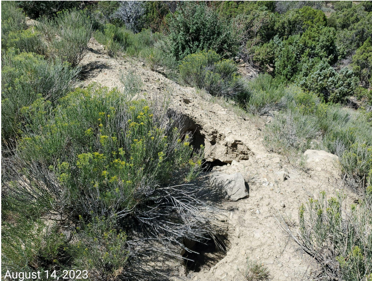
Photo 8: Photo taken from the fill slopes. Photo shows erosion degradation due to stormwater runoff.
