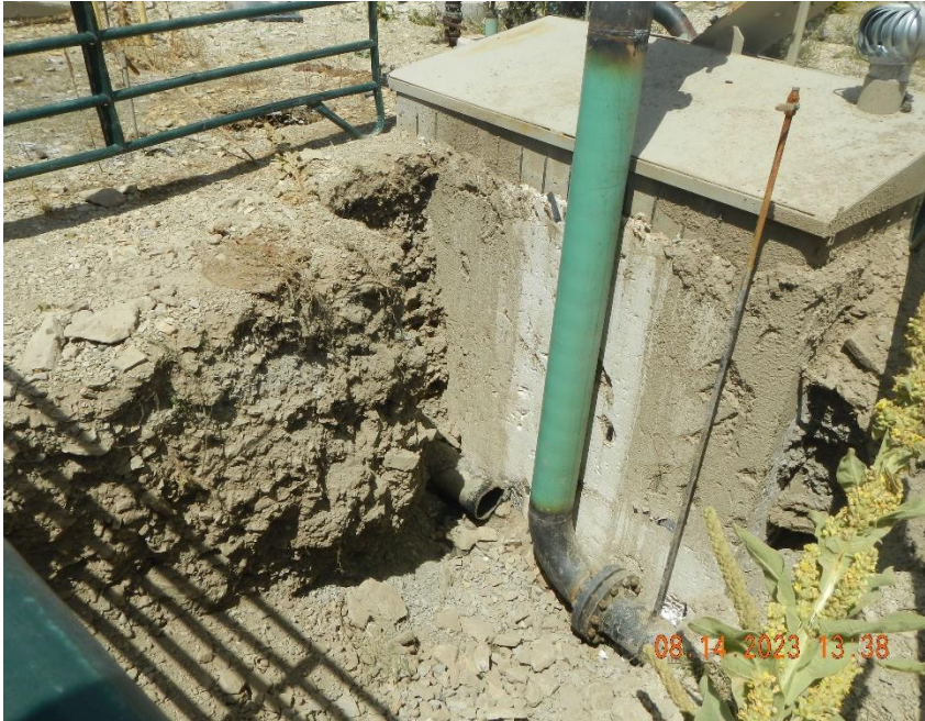
Open ended cut of 8" line in excavation.
