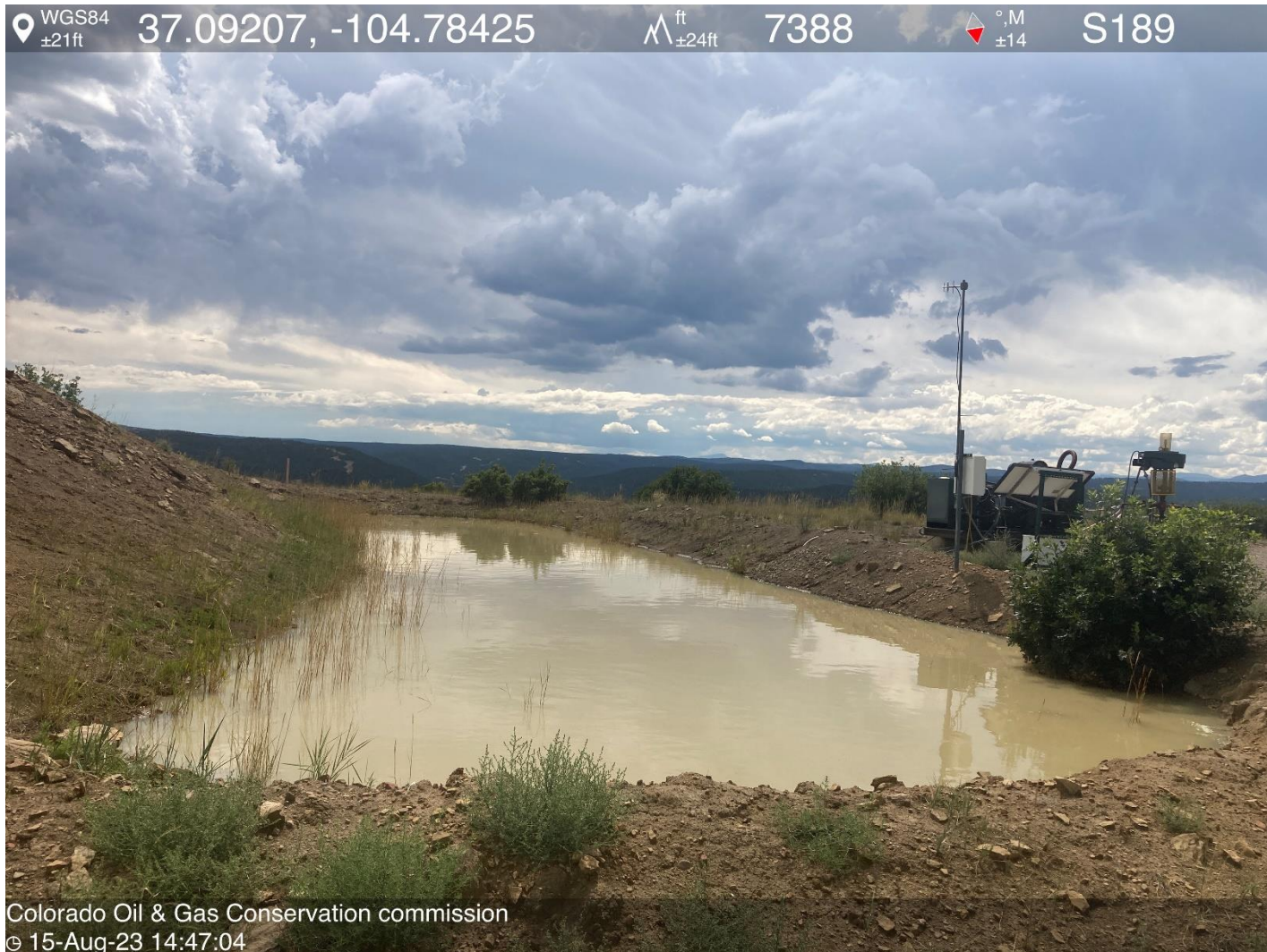
PHOTO 4: PRODUCED WATER PIT/ FLUID LEVEL IS ABOVE FREEBOARD (CONTACTED ZEKE SANCHES WITH EVERGREEN). Lower fluid level so at least two feet of freeboard exists per Rule 909.c. CA DATE 8-16-2023.
